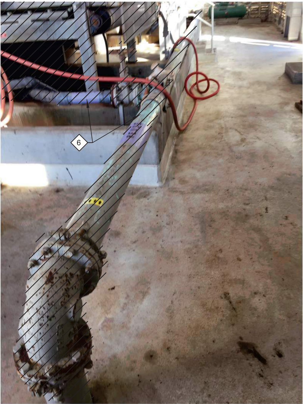
3 PHOTO SHOWING WASHWATER PIPING MD01
