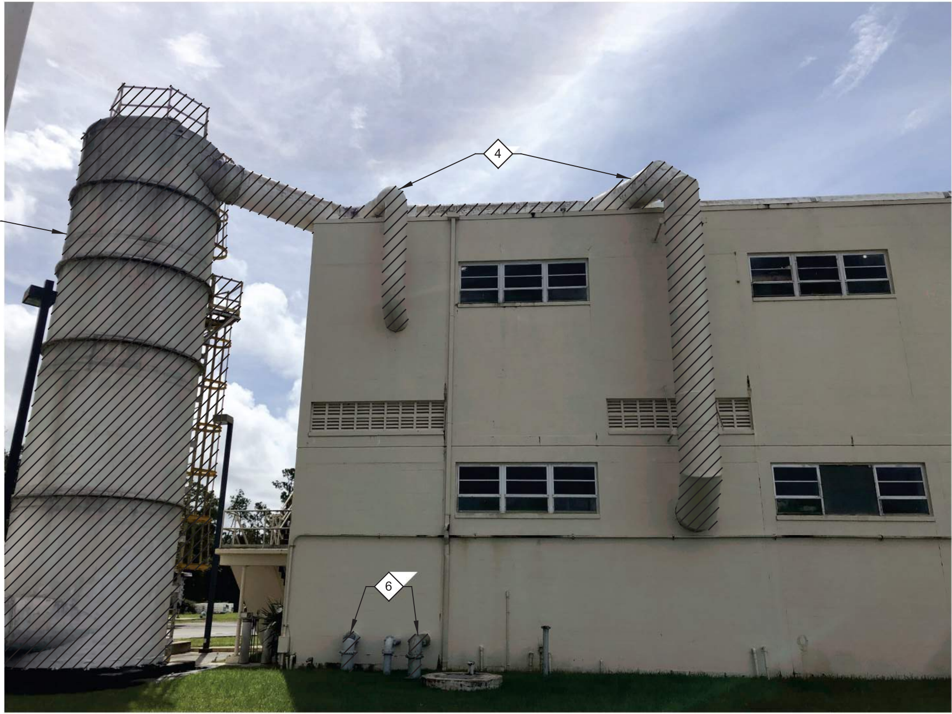
1 PHOTO SHOWING FLOCK TANK AND ODOR CONTROL DUCT
