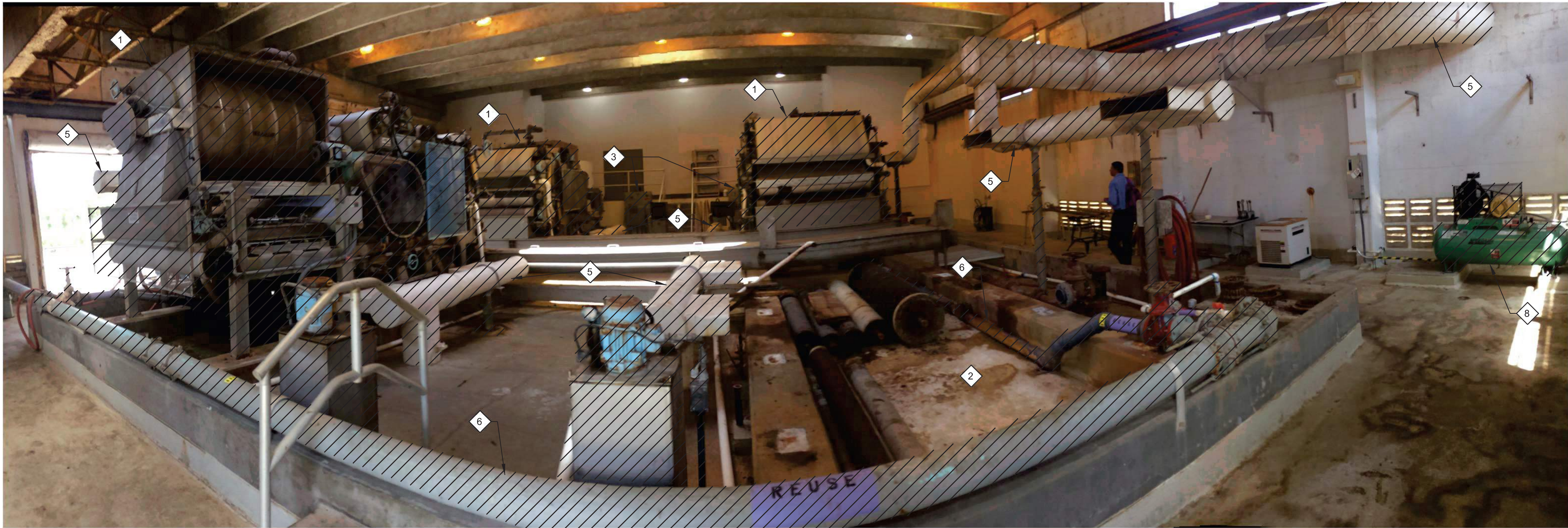
1 PHOTO SHOWING BFP No. 4, ODOR CONTROL DUCTWORK, SLDGE FEED PIPING, WASHWATER PIPING ON EAST SIDE OF DEWATERING SYSTEM MD01
