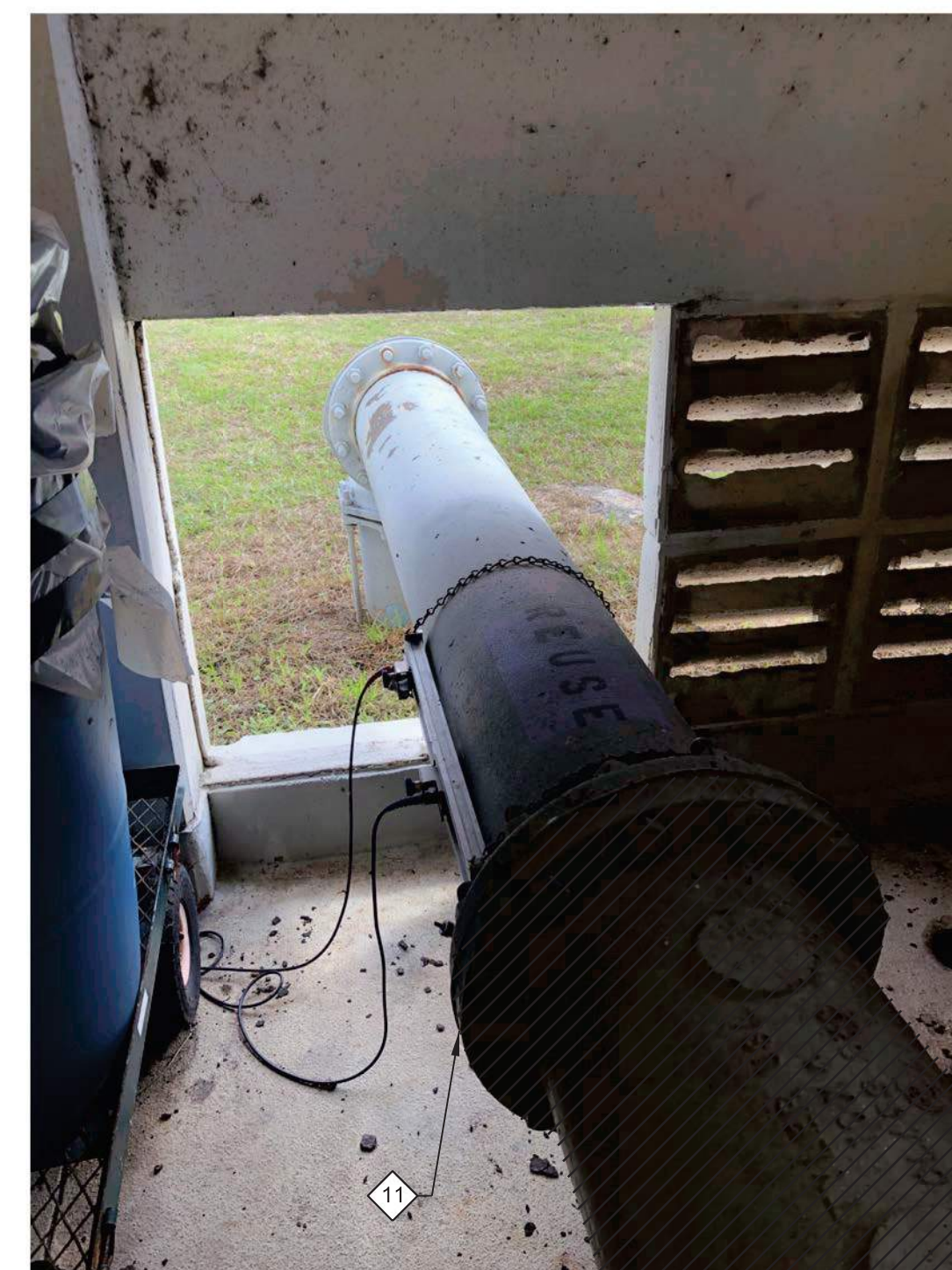
10 PHOTO SHOWING REUSE WATER 10" AT THE SOUTH EAST MD03 CORNER OF THE BUILDING
