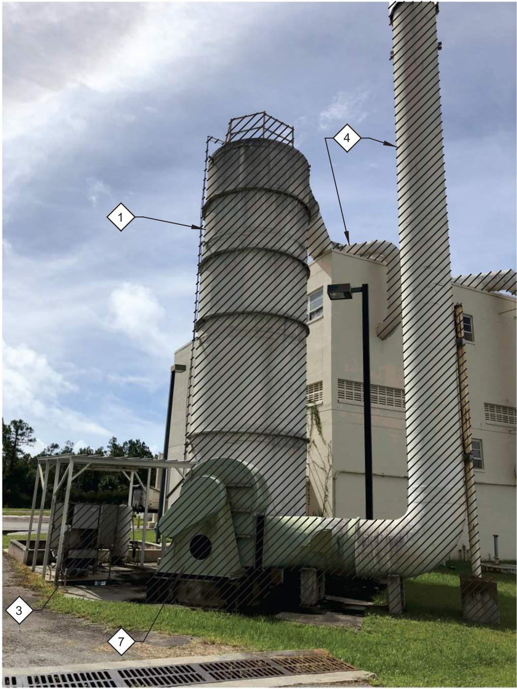
3 PHOTO SHOWING FLOCK TANK, ODOR CONTROL DUCT, AIR COMPRESSOR AND AUXILIARY EQUIPMENT
