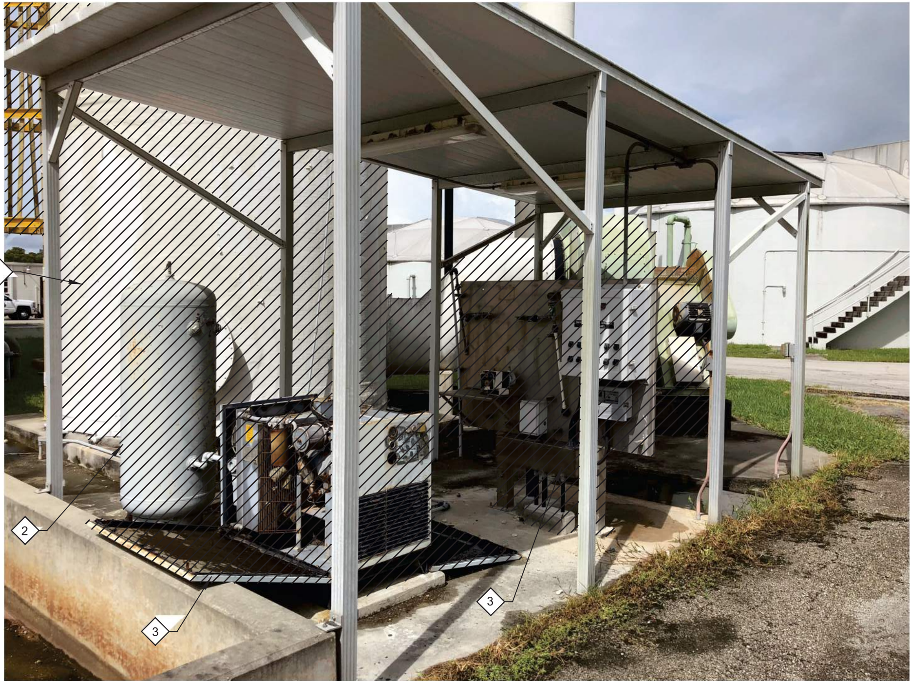
2 PHOTO SHOWING AIR COMPRESSOR AND AUXILIARY EQUIPMENT
