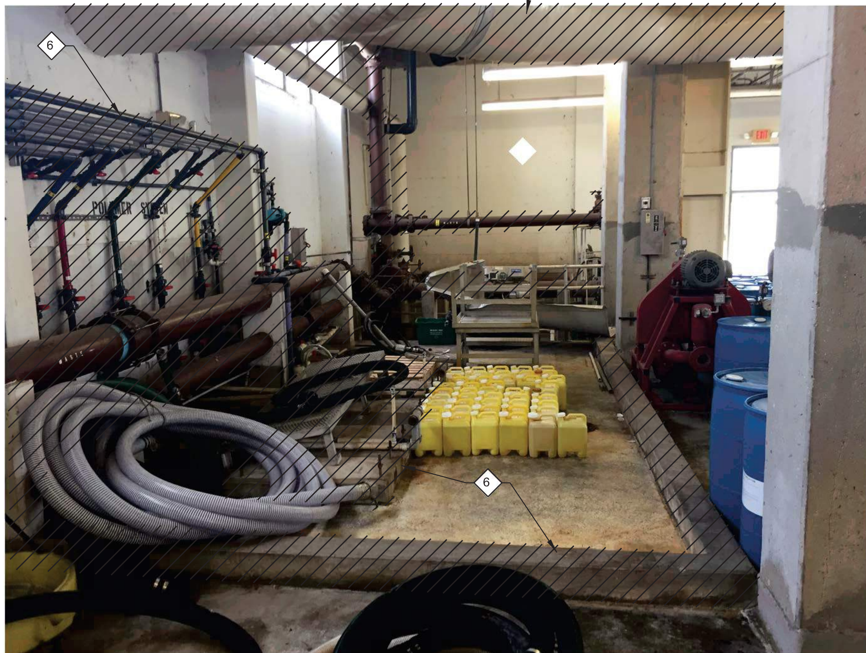
5 PHOTO SHOWING ABANDONED POLYMER SYSTEM MD03
