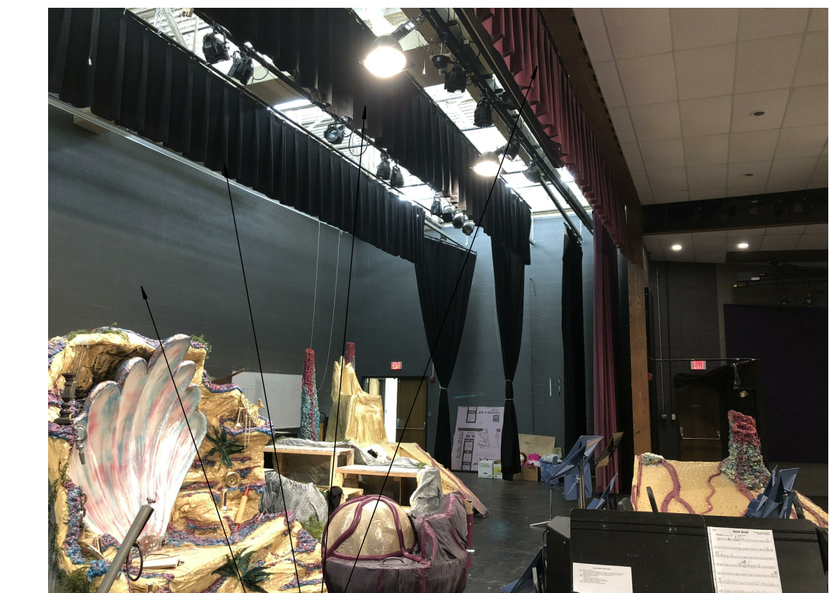
PROVIDE (N) STAGE CURTAINS THROUGHOUT. REF. SPECIFICATIONS & BID ALTERNATE #11. WALL TO BE DEMOD PER AD1.4
