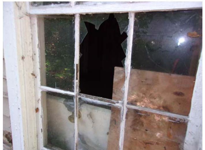
Photo 4 – Wooden windows with glazing & caulk
