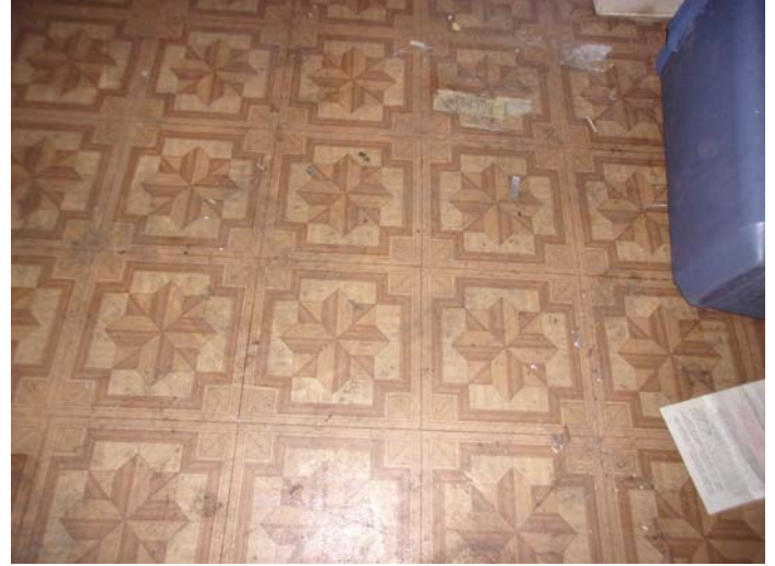
Photo 6 – 12" x 12" wooden pattern self-stick floor tiles in the kitchen & bathroom threshold
