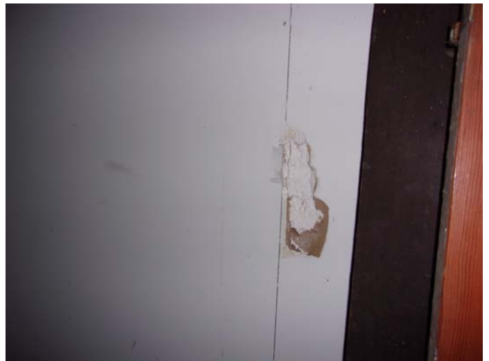
Photo 4 – Drywall with joint compound & tape throughout
