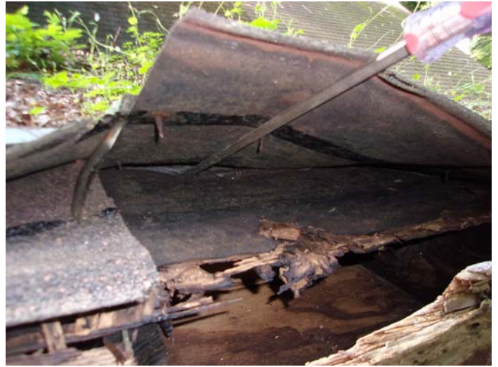
Photo 2 – Roof shingles & felt
