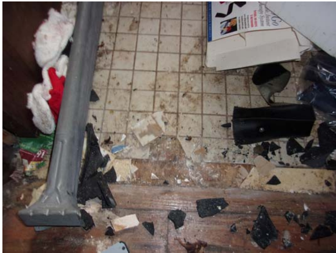
Photo 3 – Ceramic floor tile with mastic in the downstairs & upstairs bathrooms
