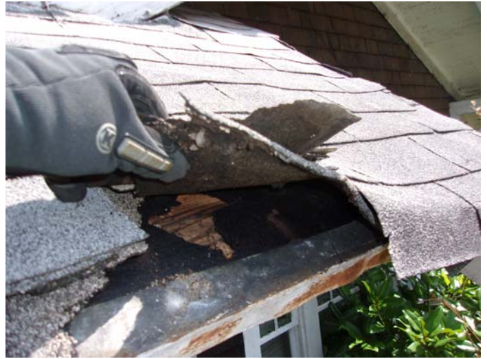
Photo 2 – Roof shingles & felt
