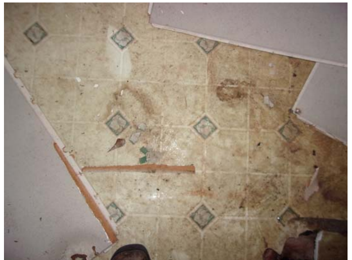
Photo 10 – Yellow square pattern roll vinyl with no mastic in the kitchen & pantry – top layer
