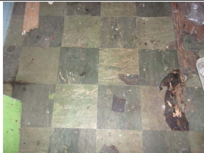
Photo 7 – 9" x 9" green/black checker pattern floor tile with mastic & felt in the right bedroom & hallway
