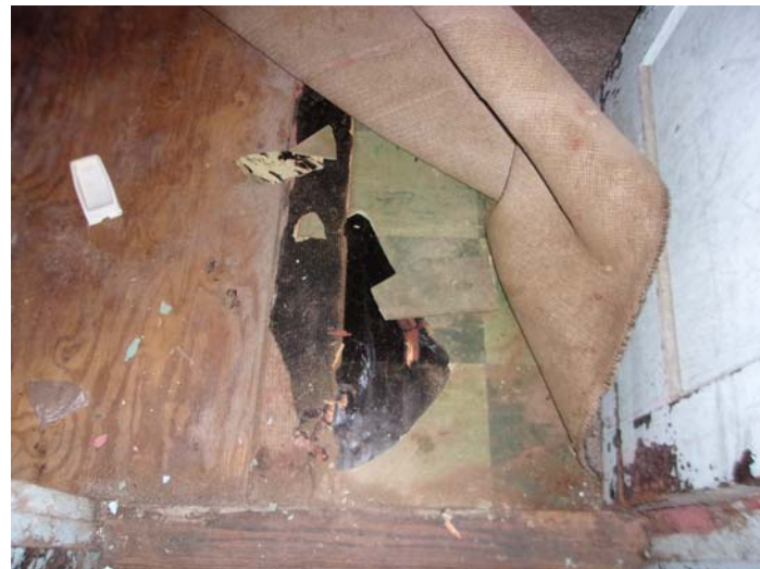
Photo 9 – 9" x 9" green & off-white checker pattern floor tiles with mastic & felt in the bathroom
