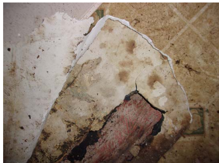
Photo 11– Tan roll vinyl floor with no mastic in the kitchen & pantry – bottom layer
