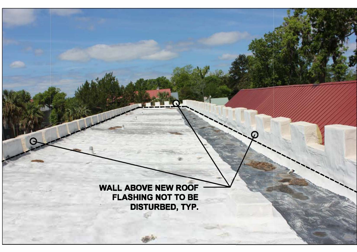
4 MUSEUM ROOF LOOKING WEST
