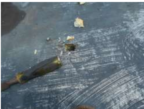
HOMOGENEOUS AREA 05 ROOF CORE (HIGH ROOF)
