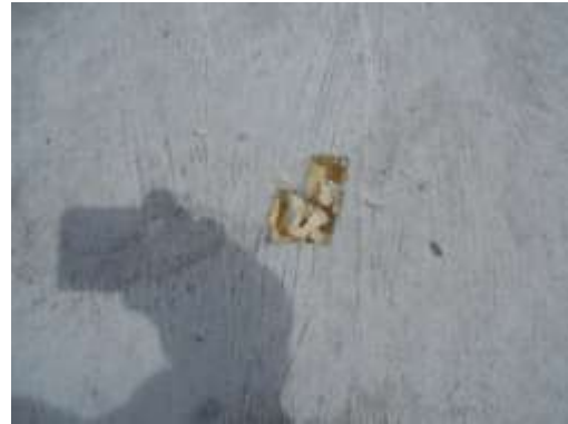
HOMOGENEOUS AREA 02 ROOF CORE (LOW ROOF)
