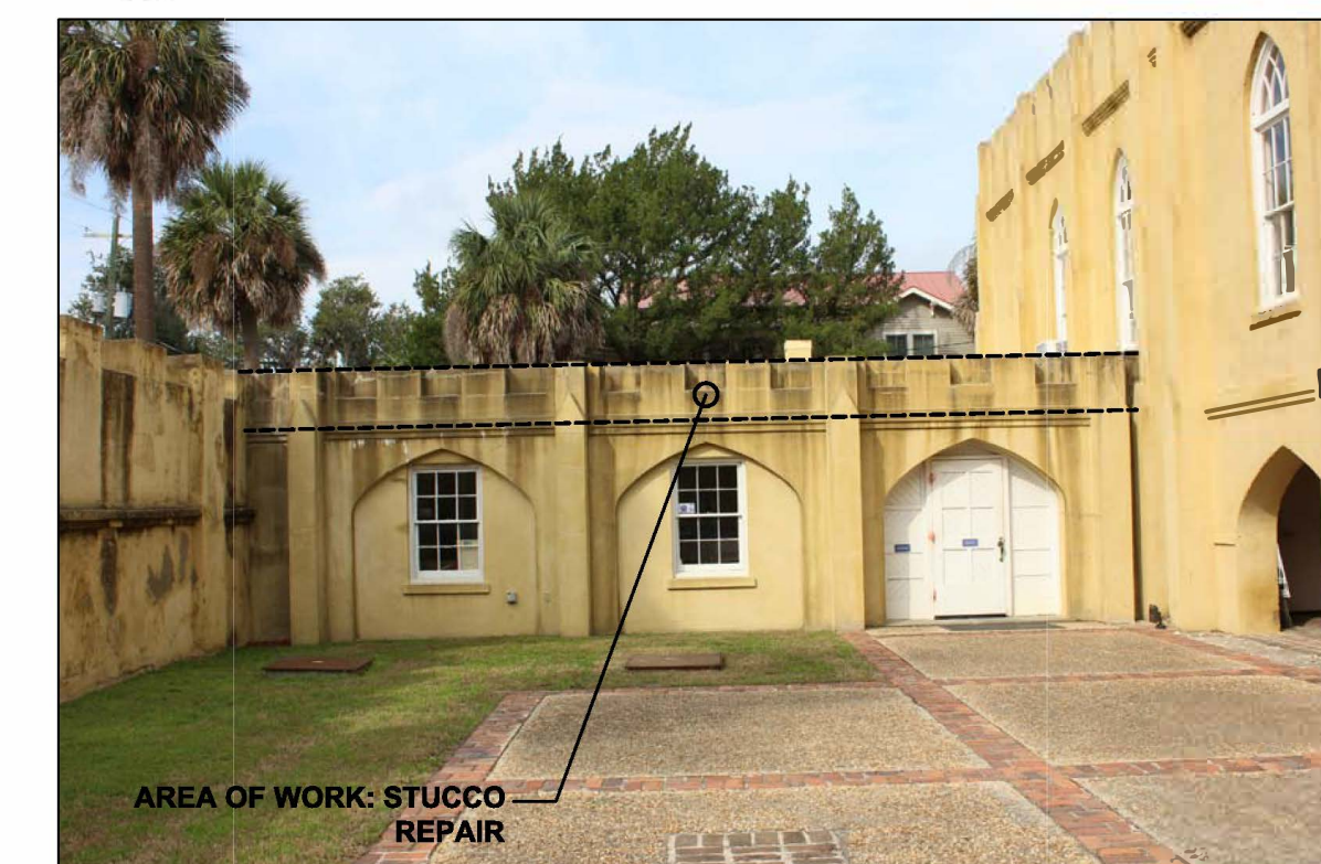
7 AREA OF WORK: STUCCO REPAIR, TYP. LOOKING WEST
