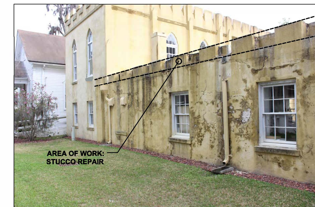
6 AREA OF WORK: STUCCO REPAIR, TYP. LOOKING WEST
