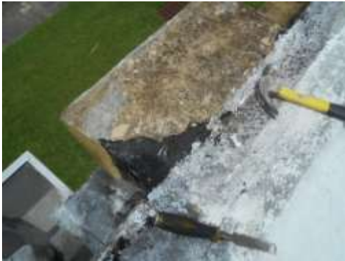
HOMOGENEOUS AREA 01 ROOF FLASHING (LOW ROOF)
