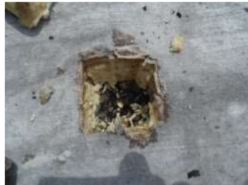
HOMOGENEOUS AREA 04 ROOF FLASHING (HIGH ROOF)
