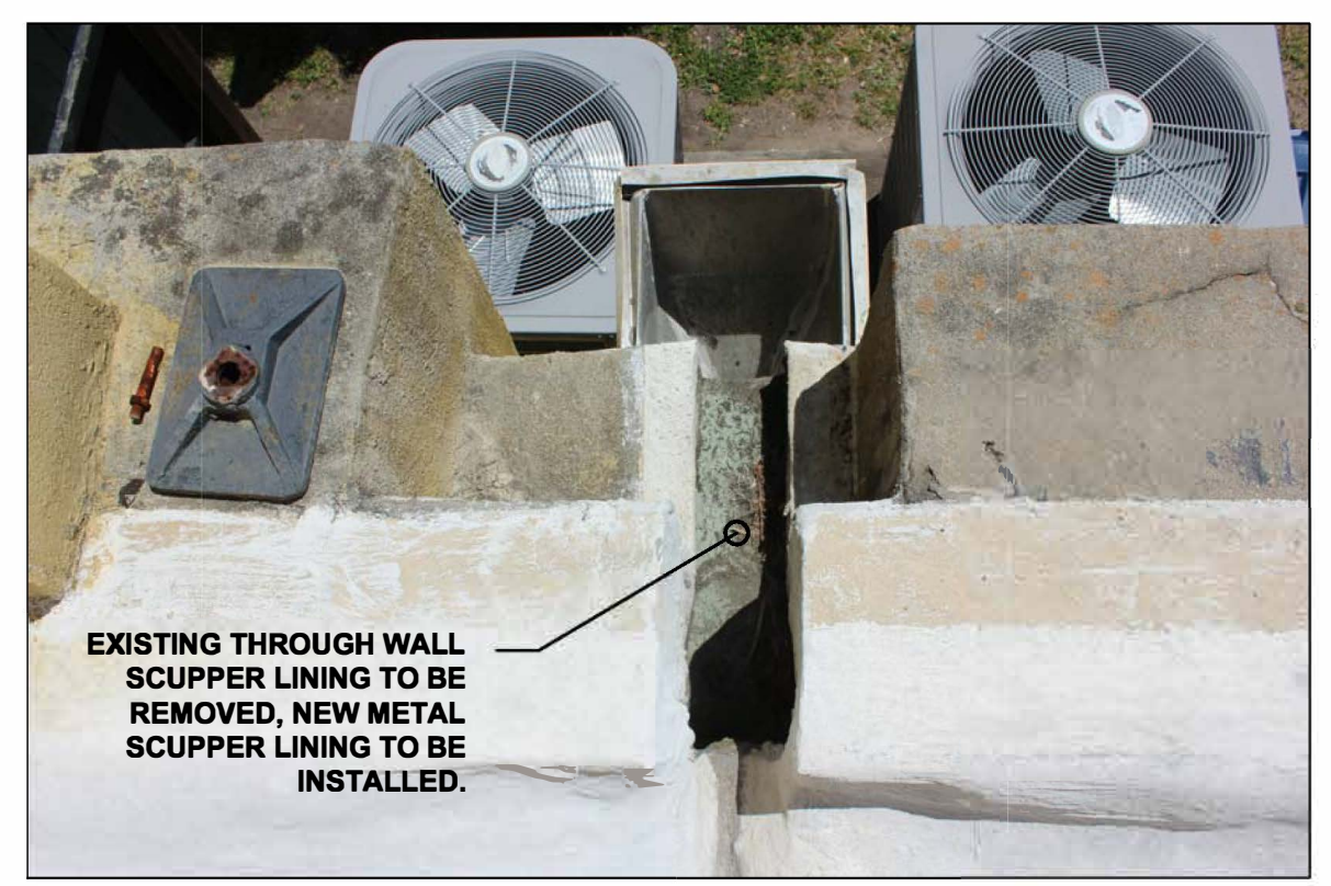
5 A101 VISITOR'S CENTER ROOF LOOKING EAST
