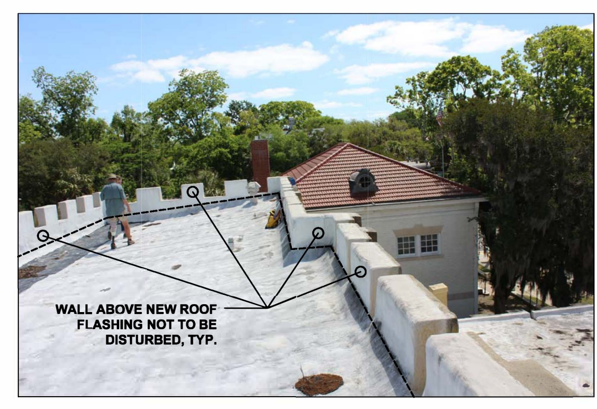
5 MUSEUM ROOF LOOKING EAST
