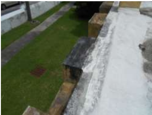
HOMOGENEOUS AREA 03 TAR APPLICATION (LOW ROOF)
