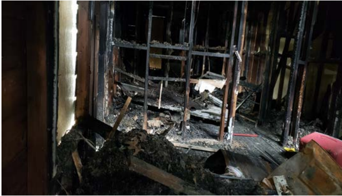
Photo 3 – Interior of residence.
