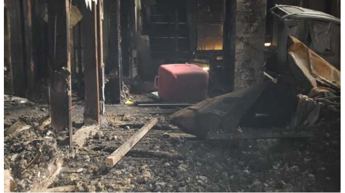
Photo 4 – Interior of residence.
