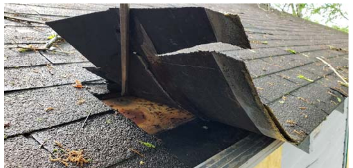
Photo 6 – Roof shingles & felt
