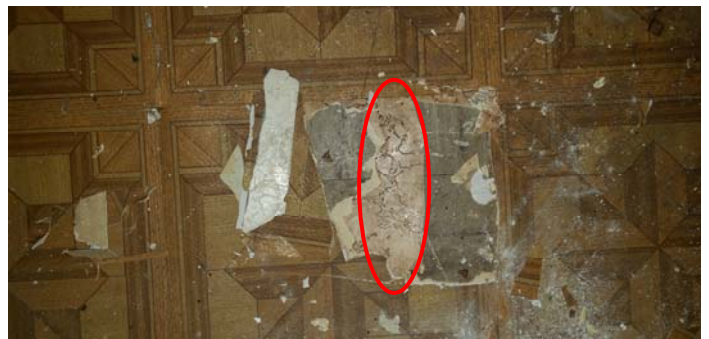
Photo 8 – Second layer of flooring in the bathroom is a tan rock fissure pattern with no mastic.
