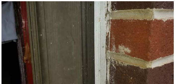
Photo 6 – Caulk located on exterior metal door frame.
