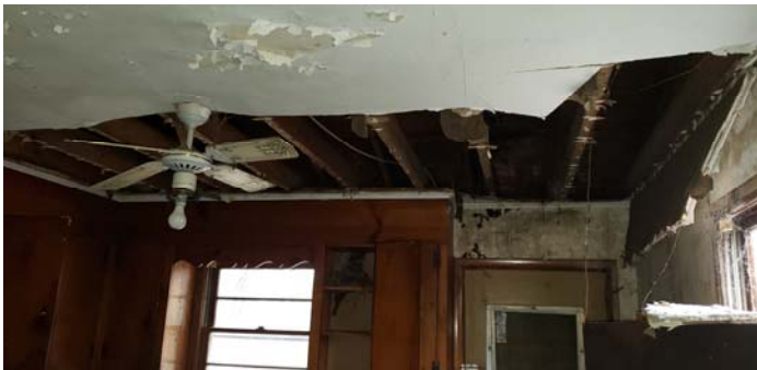
Photo 11 – Swirl ceiling texture over drywall and plaster with finish. Collapsed ceiling in areas of structure.
