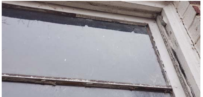
Photo 4 – Wooden windows with glazing.
