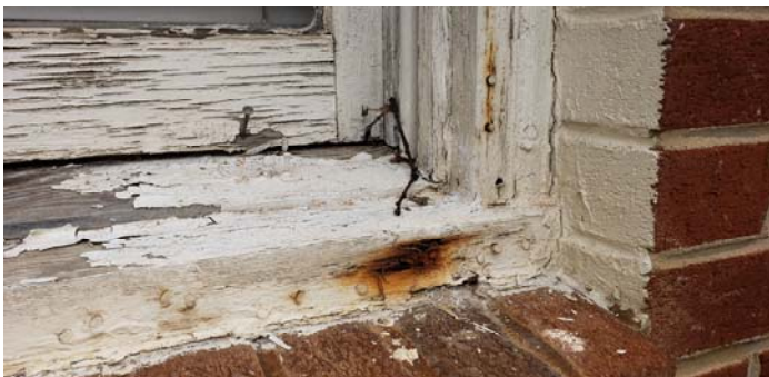
Photo 5 – Caulk located on exterior wood window frame.
