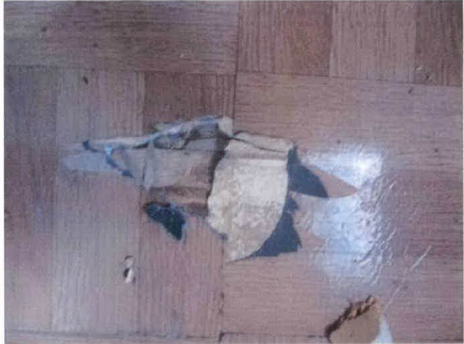
Photo 14 – 12" x 12" wooden pattern self-stick floor tile over tan vinyl floor & mastic in the bathroom (1 st & 2 nd layers)
