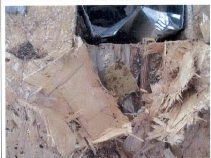
Photo 13 – 12" x 12" brown floor tile & mastic over floor tile & mastic in the kitchen (4th & 5th layers under wood)
