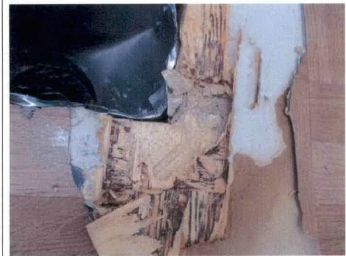
Photo 15 – Beige vinyl floor with no mastic in the bathroom (3rd layer under wood)
