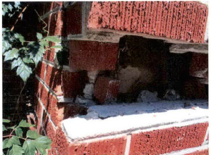
Photo 8 – Unfinished drywall throughout under brick siding
