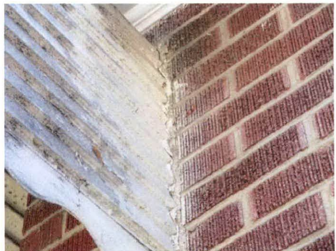
Photo 6 – Caulk/glazing on the metal awning over the front porch
