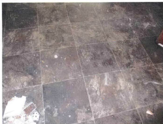
Photo 11 – Green large square pattern vinyl floor & adhesive in the kitchen & in the hallway closet (top layer)
