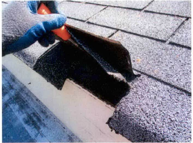
Photo 2 – Roof shingles & felt paper
