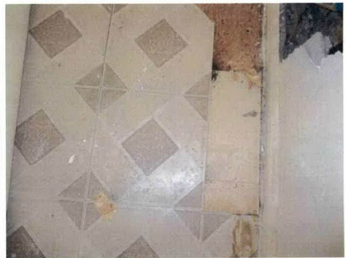
Photo 12 – 12" x 12" gray square pattern self-stick floor tile over floor tile & adhesive in the kitchen (2 nd /3 rd layers)
