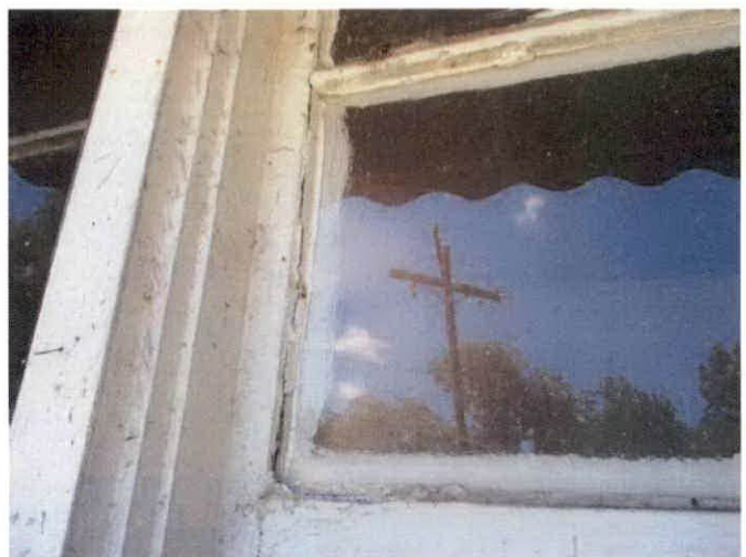
Photo 4 – Wooden window glazing
