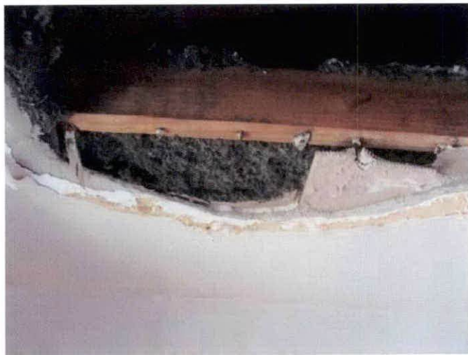
Photo 9 – Plaster with finish over unfinished drywall ceilings throughout
