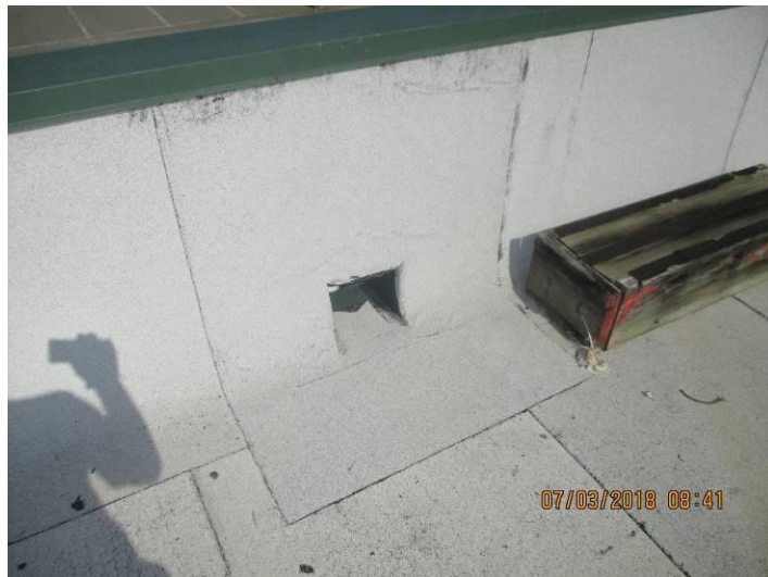
# 29: Scuppers are in good condition.
