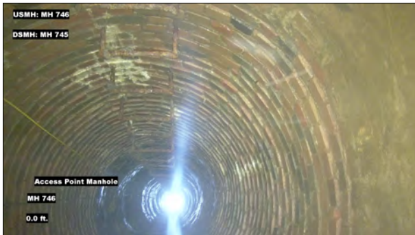
Photo: MH746_D_MH745_AMH_0.jpg, VCR No.: 1 0FT, Manhole
