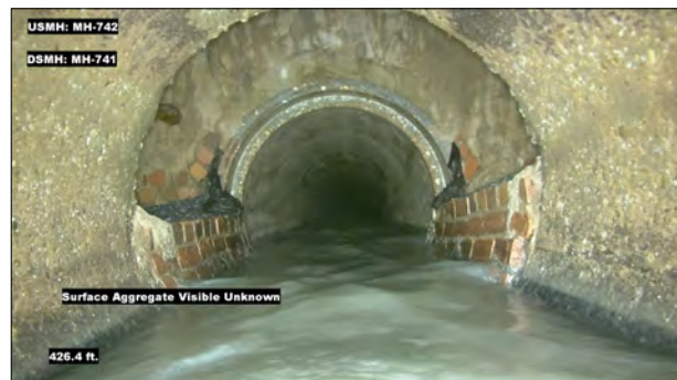
Photo: MH742_D_MH741_SAVZ_426.4.jpg, VCR No.: 1 426.4FT, Surface Aggregate Visible Unknown, from 09 to 03 o'clock, within 8 inches: NO
