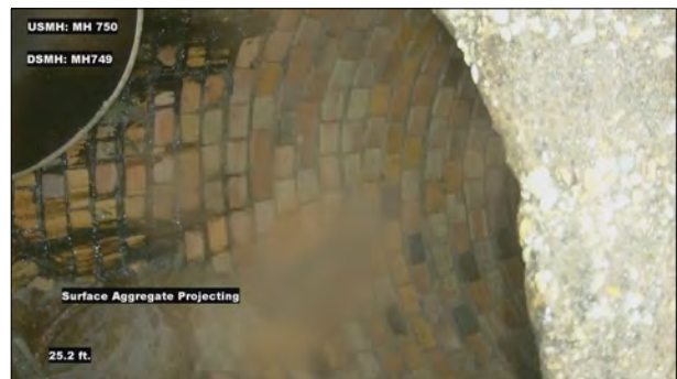
Photo: MH750_U_MH749_SAV_26.jpg, VCR No.: 1 26FT, Surface Aggregate Visible, from 09 to 03 o'clock, within 8 inches of joint: YES, Finish
