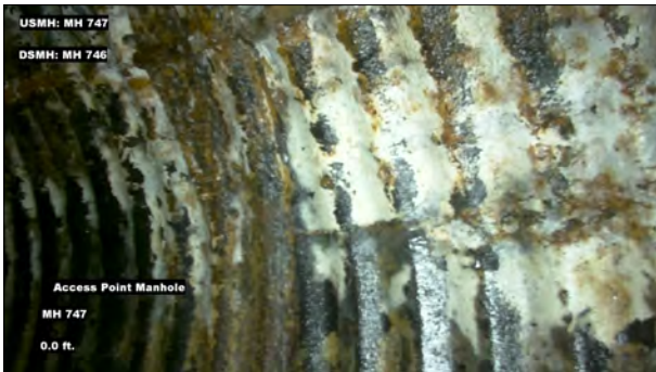
Photo: MH747_D_MH746_AMH_0.jpg, VCR No.: 1 0FT, Manhole
