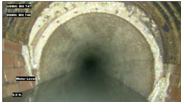
Photo: MH747_D_MH746_MWL_0.jpg, VCR No.: 1 0FT, Water Level, 15 %of cross sectional area
