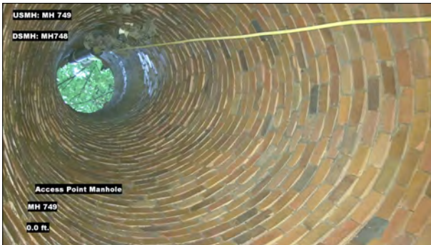
Photo: MH749_D_MH748_AMH_0.jpg, VCR No.: 1 0FT, Manhole
