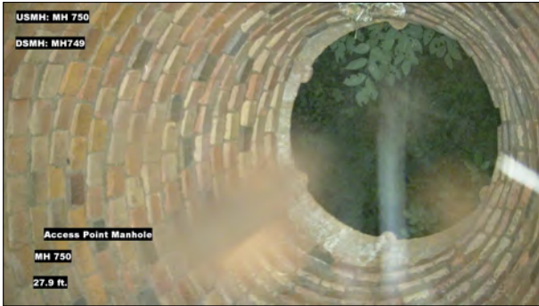
Photo: MH750_U_MH749_AMH_27.9.jpg, VCR No.: 1 27.9FT, Manhole
