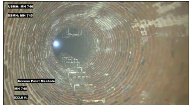
Photo: MH746_D_MH745_AMH_533.jpg, VCR No.: 1 533FT, Manhole
