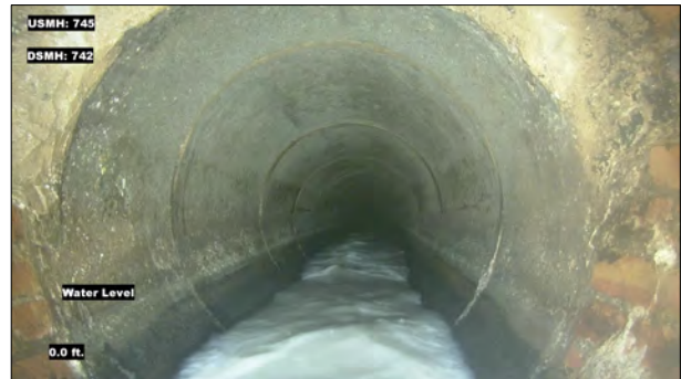
Photo: MH745_D_MH742_MWL_0.jpg, VCR No.: 1 0FT, Water Level, 5% of cross sectional area
