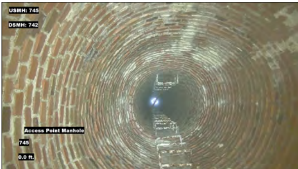
Photo: MH745_D_MH742_AMH_0.jpg, VCR No.: 1 0FT, Manhole
