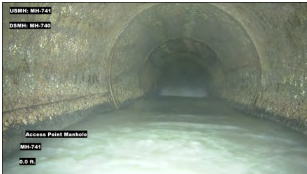
Photo: MH741_D_MH740_AMH_0.jpg, VCR No.: 1 0FT, Manhole
