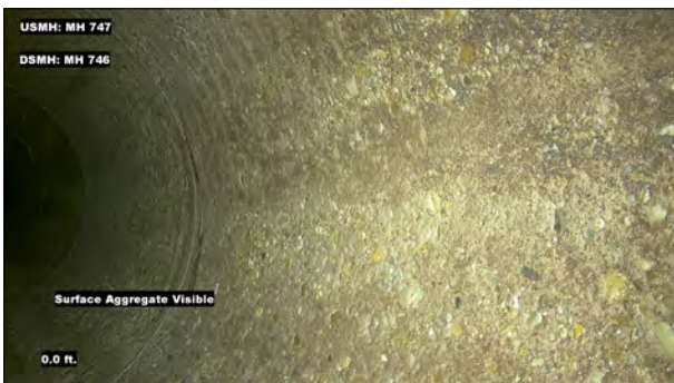
Photo: MH747_D_MH746_SAV_0.jpg, VCR No.: 1 0FT, Surface Aggregate Visible, from 07 to 05 o'clock, within 8 inches: YES
