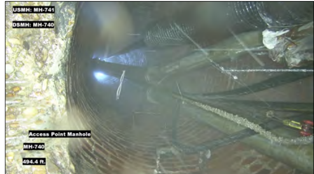
Photo: MH741_D_MH740_AMH_494.4.jpg, VCR No.: 1 494.4FT, Manhole
