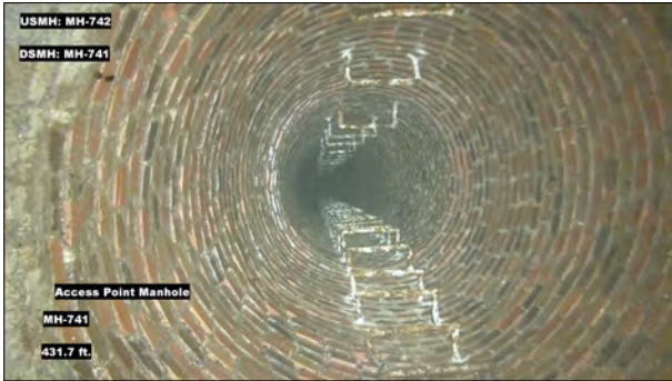
Photo: MH742_D_MH741_AMH_431.7.jpg, VCR No.: 1 431.7FT, Manhole
