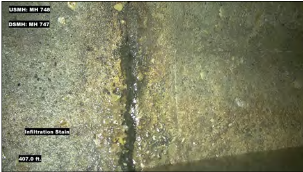
Photo: MH748_D_MH747_IS_407.jpg, VCR No.: 1 407FT, Infiltration Stain, from 07 to 08 o'clock, within 8 inches: NO
