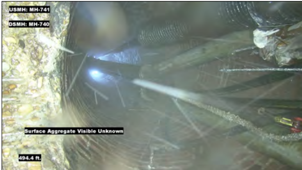
Photo: MH741_D_MH740_SAVZ_494.4.jpg, VCR No.: 1 494.4FT, Surface Aggregate Visible Unknown, from 08 to 04 o'clock, within 8 inches: NO
