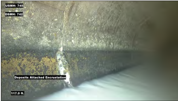
Photo: MH745_D_MH742_DAE_117.jpg, VCR No.: 1 117FT, Deposits Attached Encrustation, 5% of cross sectional area, at 08 o'clock, within 8 inches: YES
