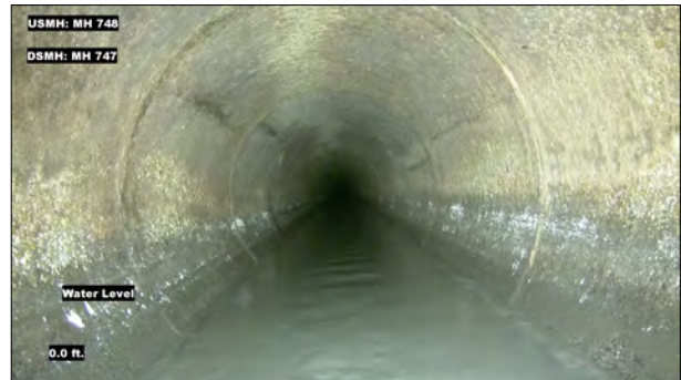
Photo: MH748_D_MH747_MWL_0.jpg, VCR No.: 1 0FT, Water Level, 10% of cross sectional area
