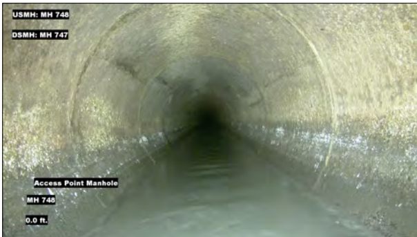
Photo: MH748_D_MH747_AMH_0.jpg, VCR No.: 1 0FT, Manhole
