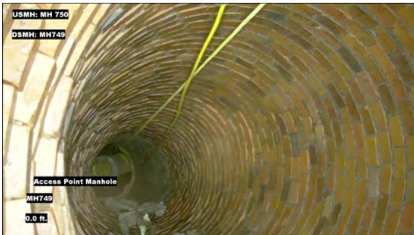
Photo: MH750_U_MH749_AMH_0.jpg, VCR No.: 1 0FT, Manhole
