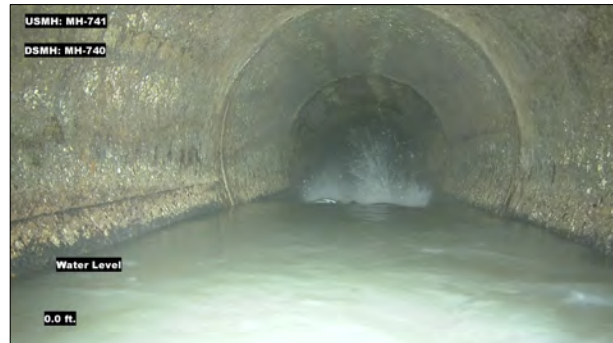
Photo: MH741_D_MH740_MWL_0.jpg, VCR No.: 1 0FT, Water Level, 10% of cross sectional area
