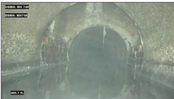
Photo: MH749_D_MH748_SAV_491.jpg, VCR No.: 1 491FT, Surface Aggregate Visible, from 09 to 03 o'clock, within 8 inches of joint: NO, Finish
