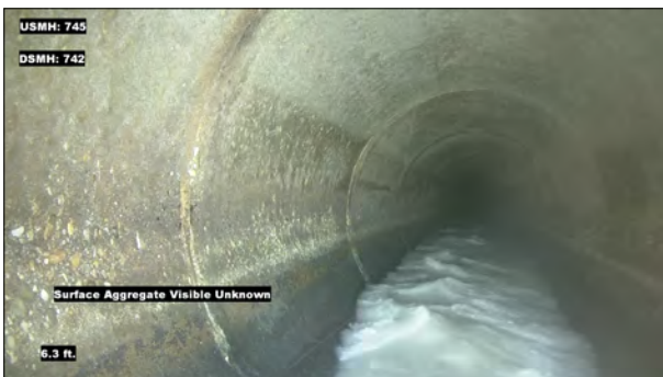
Photo: MH745_D_MH742_SAVZ_6.3.jpg, VCR No.: 1 6.3FT, Surface Aggregate Visible Unknown, from 09 to 03 o'clock, within 8 inches: NO
