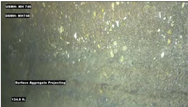
Photo: MH749_D_MH748_SAP_134.8.jpg, VCR No.: 1 134.8FT, Surface Aggregate Projecting, from 07 to 05 o'clock, within 8 inches: NO
