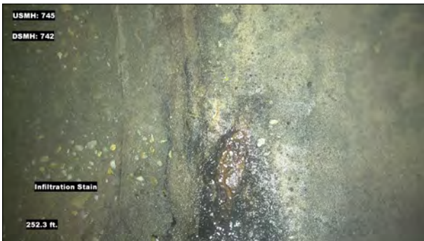
Photo: MH745_D_MH742_IS_252.3.jpg, VCR No.: 1 252.3FT, Infiltration Stain, at 03 o'clock, within 8 inches: YES
