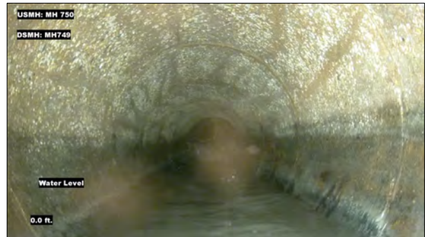
Photo: MH750_U_MH749_MWL_0.jpg, VCR No.: 1 0FT, Water Level, 10% of cross sectional area
