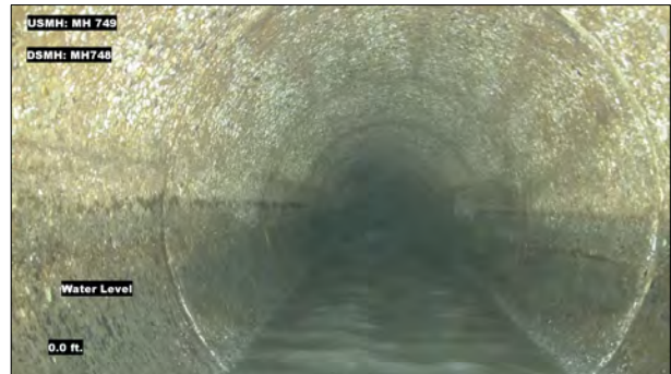
Photo: MH749_D_MH748_MWL_0.jpg, VCR No.: 1 0FT, Water Level, 10 %of cross sectional area
