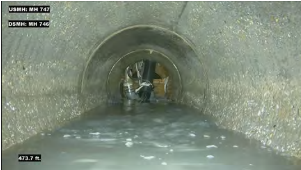
Photo: MH747_D_MH746_SAV_474.jpg, VCR No.: 1 474FT, Surface Aggregate Visible, from 07 to 05 o'clock, within 8 inches of joint: YES, Finish
