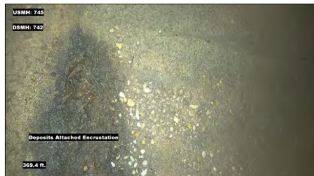
Photo: MH745_D_MH742_DAE_369.4.jpg, VCR No.: 1 369.4FT, Deposits Attached Encrustation, 5% of cross sectional area, at 11 o'clock, within 8 inches: YES
