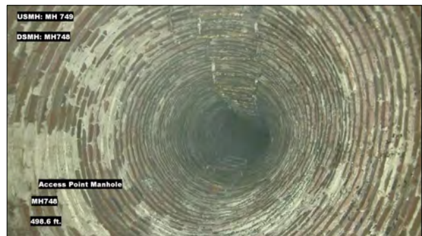
Photo: MH749_D_MH748_AMH_498.6.jpg, VCR No.: 1 498.6FT, Manhole
