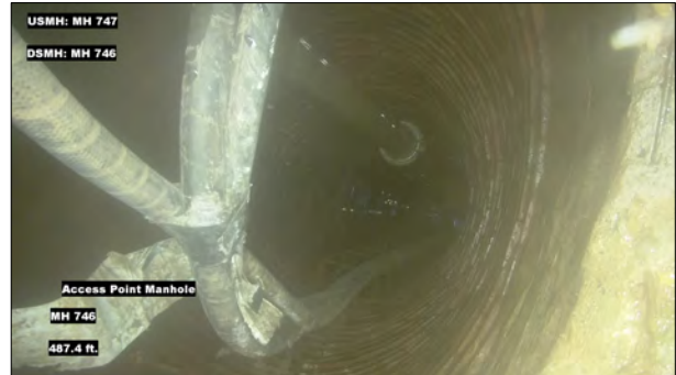
Photo: MH747_D_MH746_AMH_487.4.jpg, VCR No.: 1 487.4FT, Manhole
