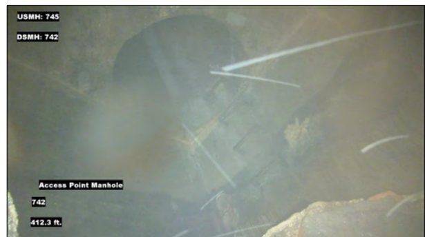
Photo: MH745_D_MH742_AMH_412.3.jpg, VCR No.: 1 412.3FT, Manhole
