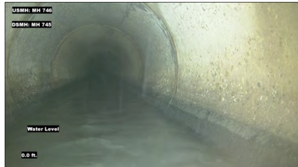
Photo: MH746_D_MH745_MWL_0.jpg, VCR No.: 1 0FT, Water Level, 5% of cross sectional area
