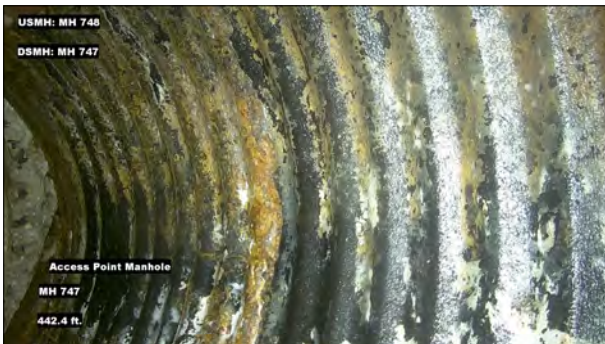
Photo: MH748_D_MH747_AMH_442.4.jpg, VCR No.: 1 442.4FT, Manhole
