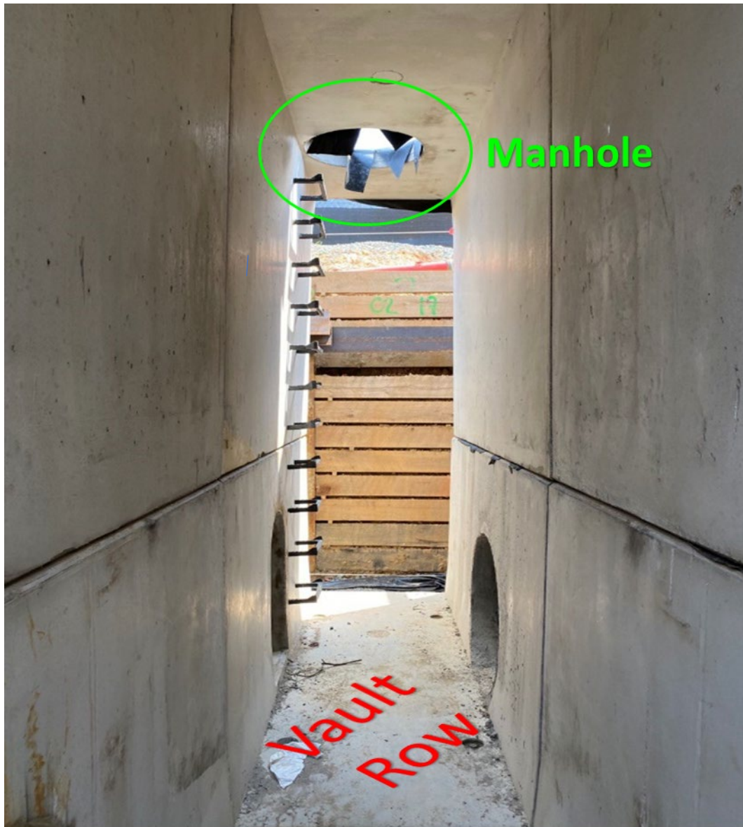
Figure 4. The underground detention vault access manhole
