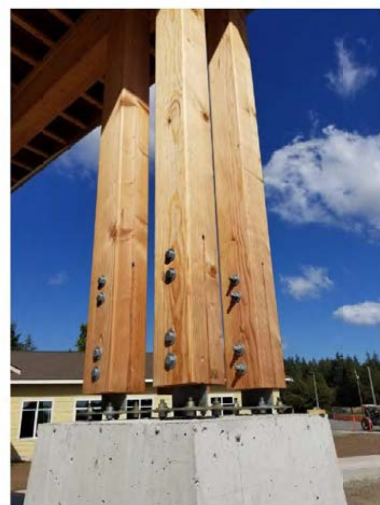
KNIFE PLATE WITH LEVELING BOLT
