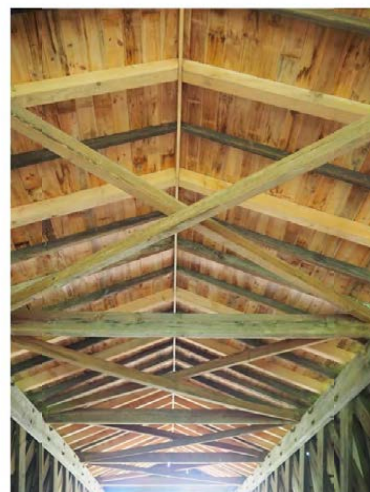
EXPOSED CEILING STRUCTURE
