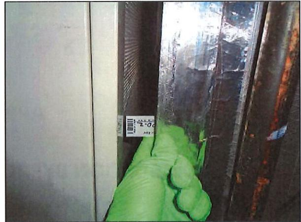
Figure (22) – Police Department HVAC Unit #2 Tape Lift Sample #PD-2 from Return Air System
