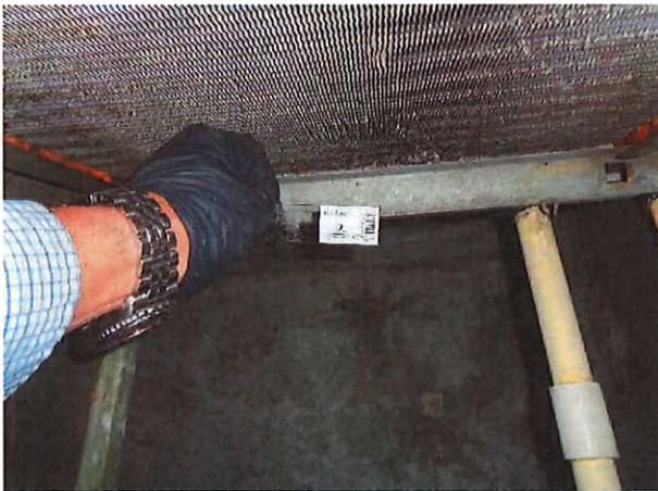
Figure (27) – #2 Tape Lift Sample from #1 HVAC Return
