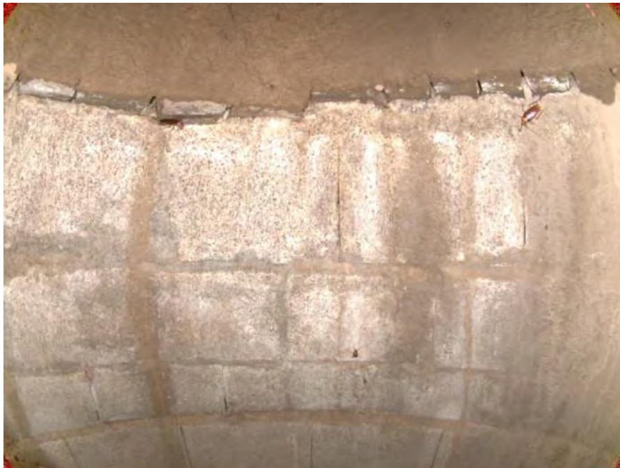
1841a_7e3e94ed-5602-4c81-88a8-bfb0bb428782_49b19cba-c025-49c9-8b0e-801e87cd9422_P11.jpg, 00:00:13, 2.38 Missing Mortar Large from 12 o'clock to 11 o'clock, Start
