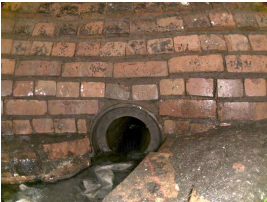
2193c_2b27c63e-1844-43c6-8c49-44849fa40c9a_ca3636fc-c371-4c76-a7b1-b6d39cd72e45_P11.jpg, 00:00:17, 3.75 Deposits Settled Fine, 5% of cross sectional area from 12 o'clock to 12 o'clock, within 8 inch
