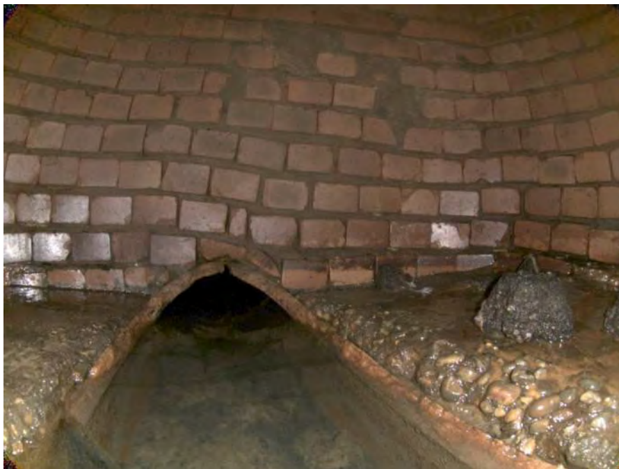
1831_511dce6f-34cf-4134-8589-97e8cd9b2803_26edafcf-9755-414d-ac9d-c19aa6e5a345_PI1.jpg, 00:00:33, 7.29 Surface Damage Aggregate Projecting from 11 o'clock to 2 o'clock, within 8 inch, Start
