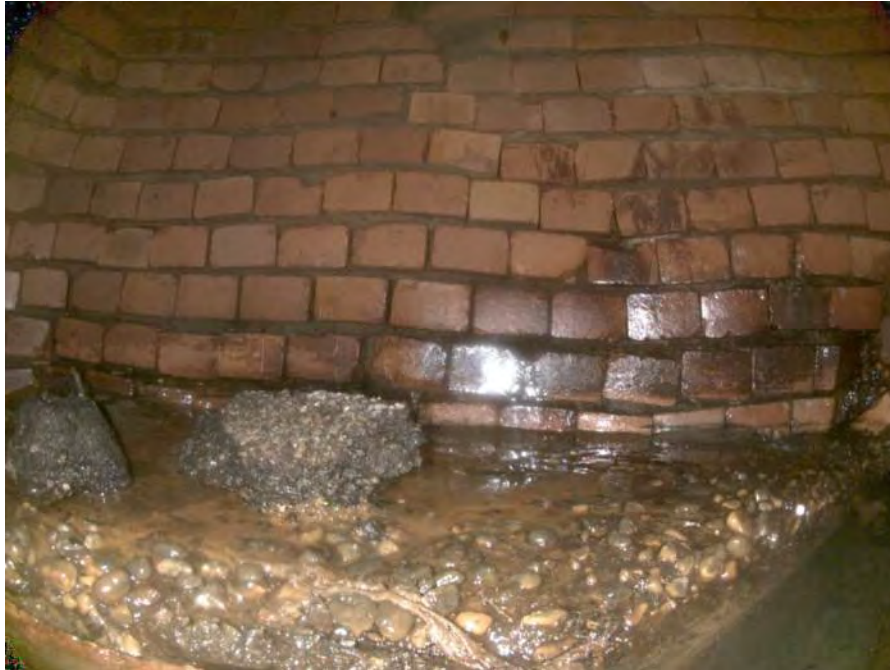
1831_511dce6f-34cf-4134-8589-97e8cd9b2803_f6d5ccc0-e1d8-4e3e-8fe5-b6471e9965fe_PI1.jpg, 00:00:33, 7.05 Obstruction Construction Debris, 5% of cross sectional area from 1 o'clock to 4 o'clock
