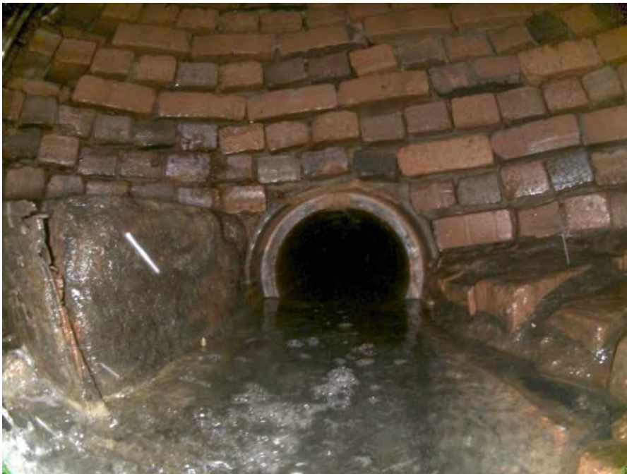
1829b_c3bb5419-4fc2-49bd-9cbb-ae8a522c6251_fafdea7a-ceca-49f8-a0fe-aca9e9443519_P11.jpg, 00:00:43, 10.53 Infiltration Dripper from 12 o'clock to 12 o'clock, within 8 inch
