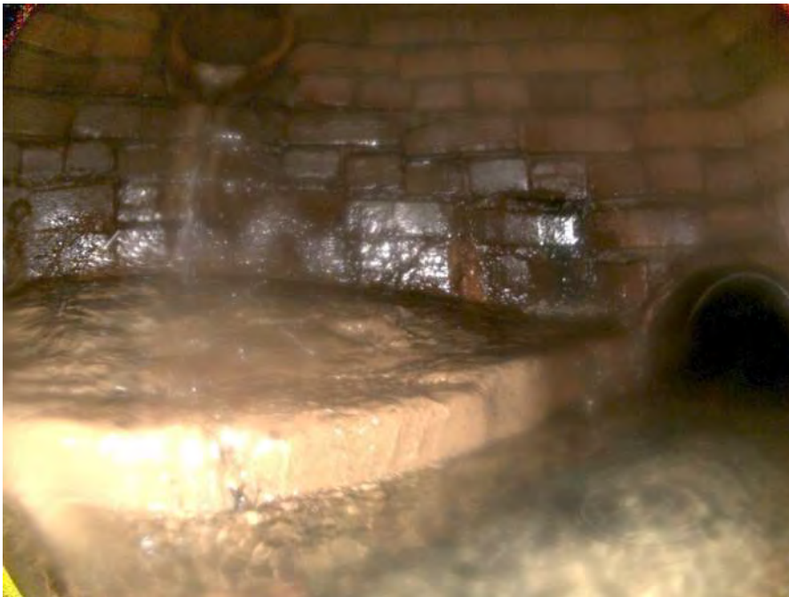
1830_f8e692ed-45a5-4111-be6d-dbb6437dd8b2_3adc60c1-ed59-466f-9d64-e0d2b984441e_PI1.jpg, 00:00:40, 8.48 Obstruction Construction Debris, 35% of cross sectional area from 1 o'clock to 10 o'clock
