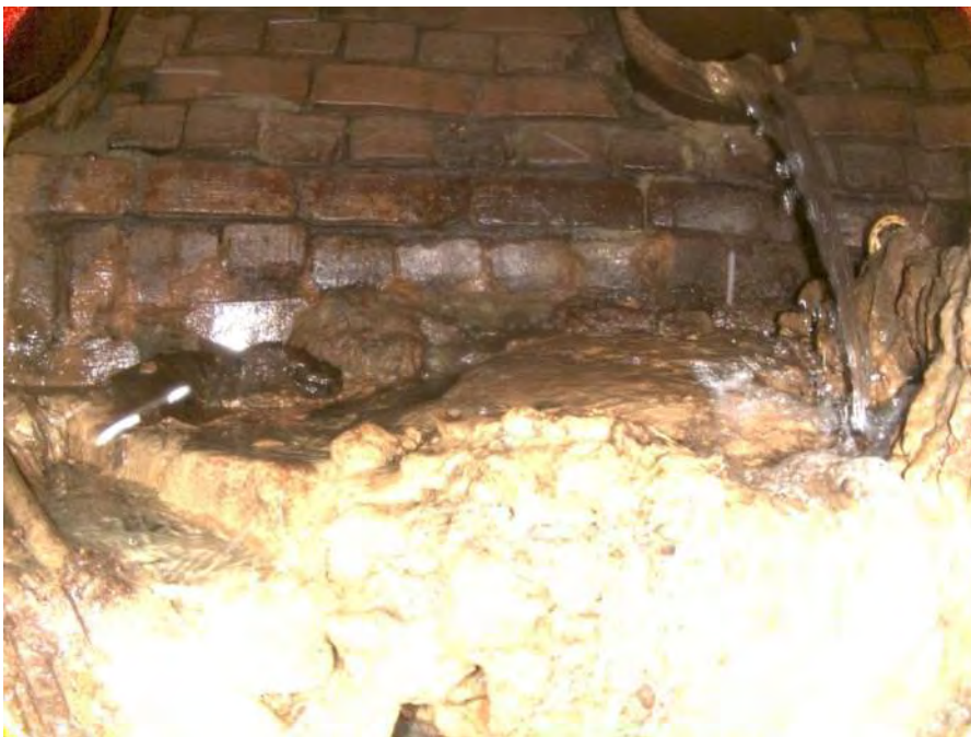
1834b_16edcb0d-7f2c-4b5a-bd27-6b0d1bf9d1bd_e218bb93-14c1-4f86-9c8f-5284944152be_P11.jpg, 00:00:34, 8.00 Obstruction Construction Debris, 30% of cross sectional area from 10 o'clock to 5 o'clock
