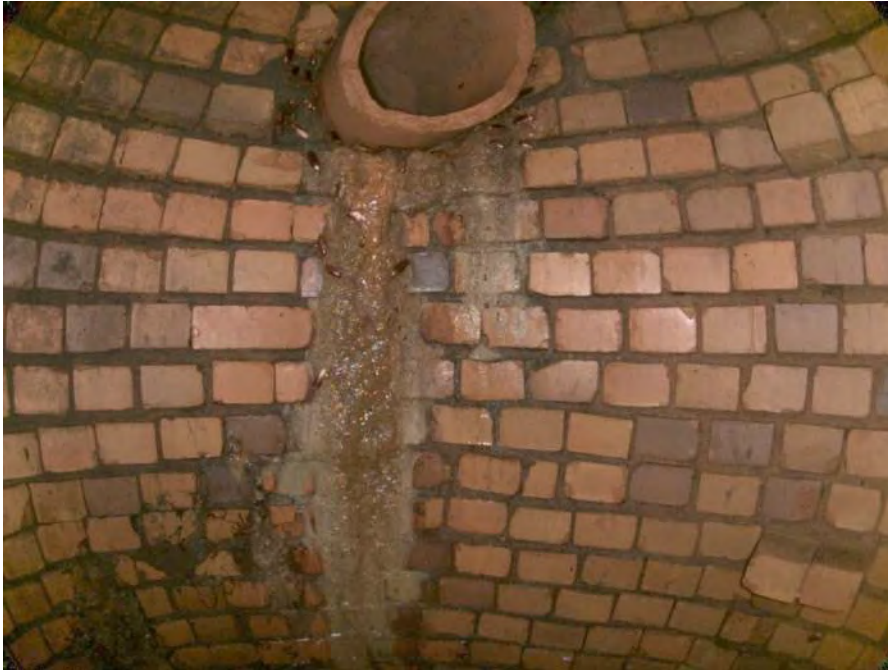
1818_a75925b2-5868-48ca-b1fe-f6e0ecc4562_5ad39124-75a8-4790-880a-2cad4d512614_P11.jpg, 00:00:27, 6.17 Infiltration Dripper from 12 o'clock to 2 o'clock, within 8 inch
