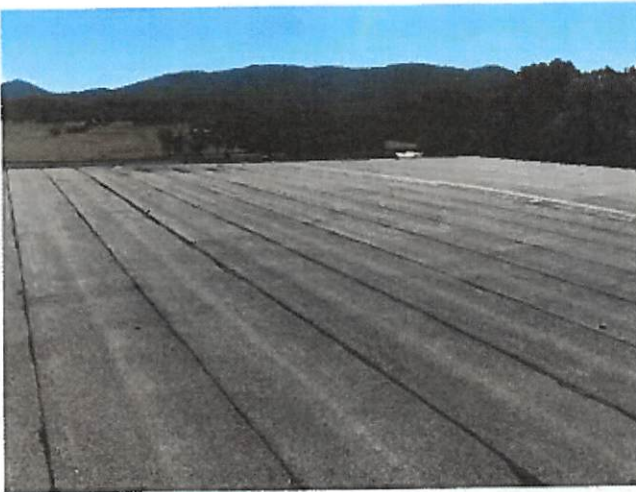
Upper roof section overview.
