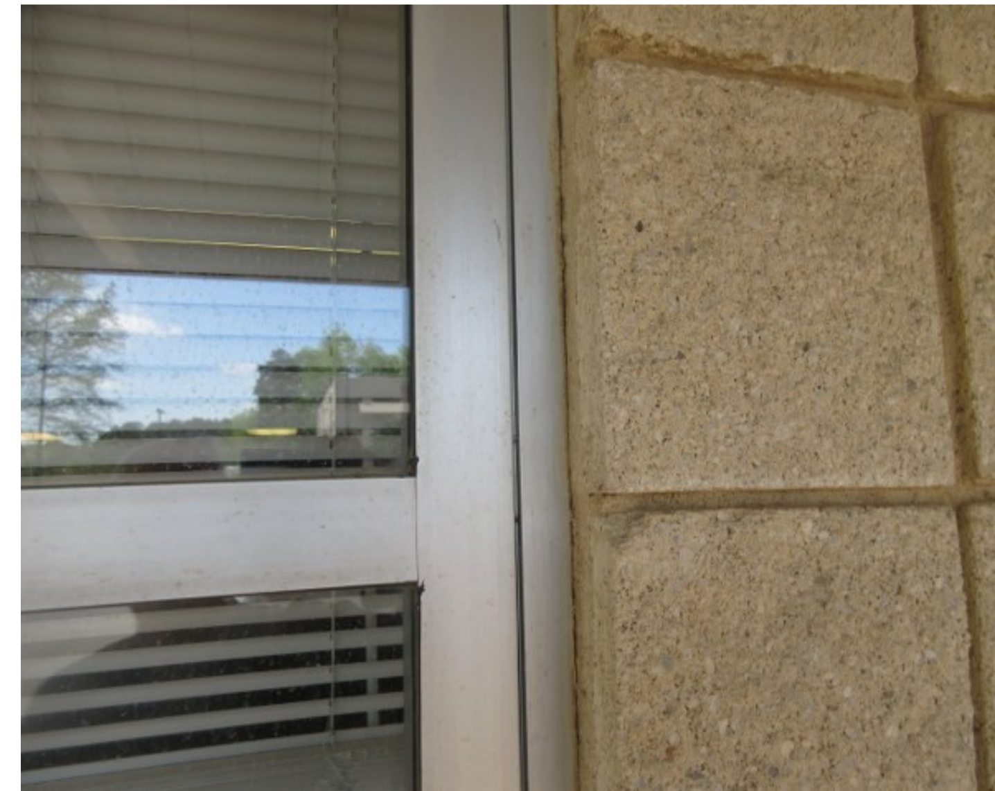
Several of the doors on the buildings have no room for a sealant joint. These areas are to be cut back to allow for a 5/8" sealant joint to be installed around the doors.
