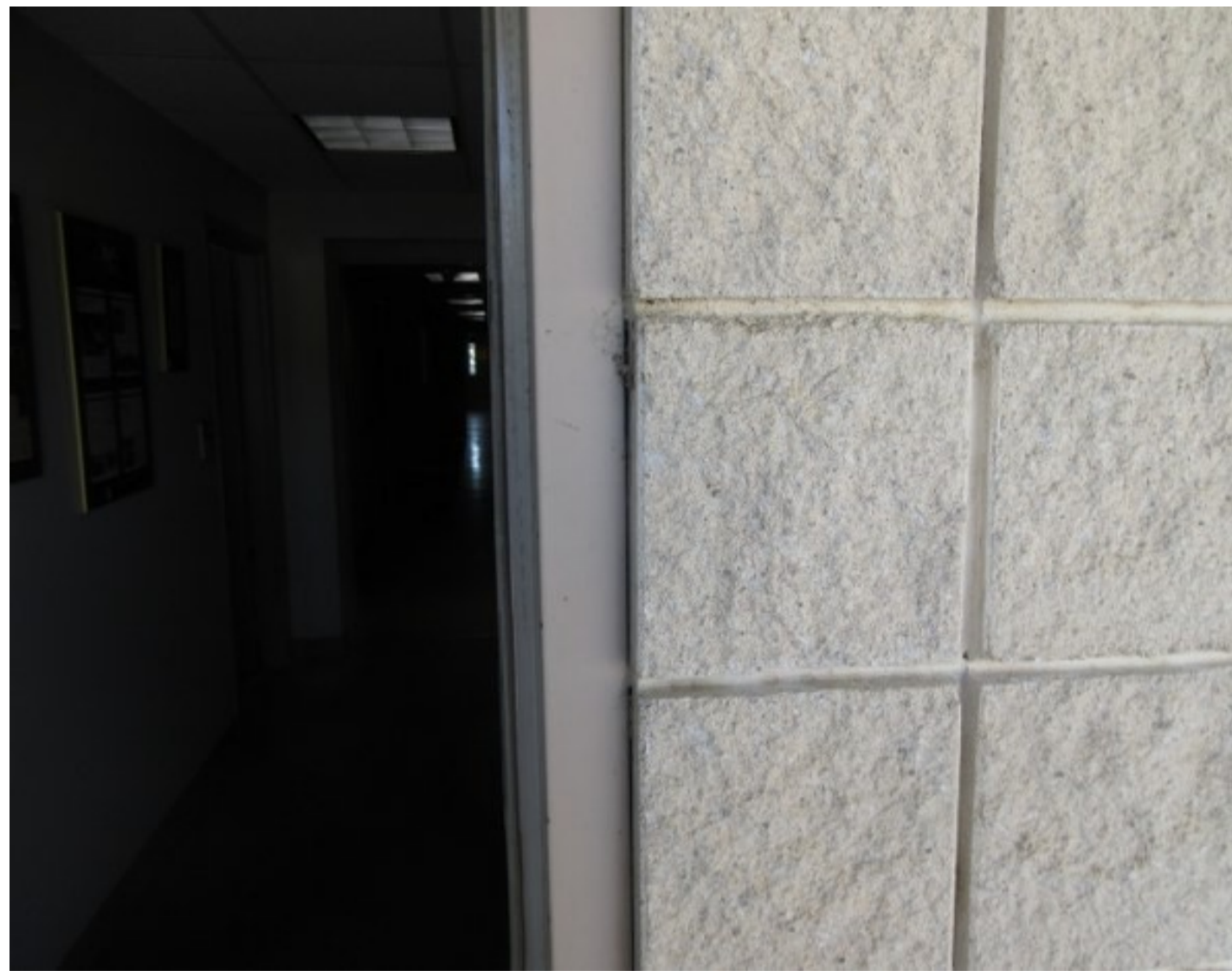
Several of the doors on the buildings have no room for a sealant joint. These areas are to be cut back to allow for a 5/8" sealant joint to be installed around the doors.
