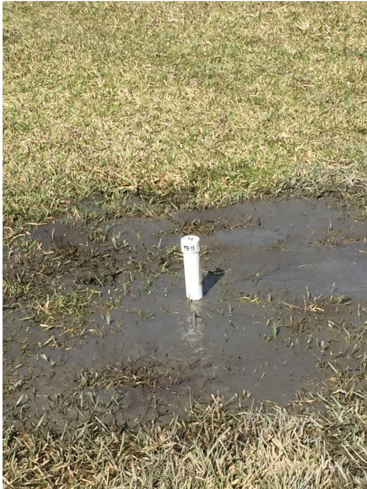
Completed SPT boring (typ.), marked for later surveying.
