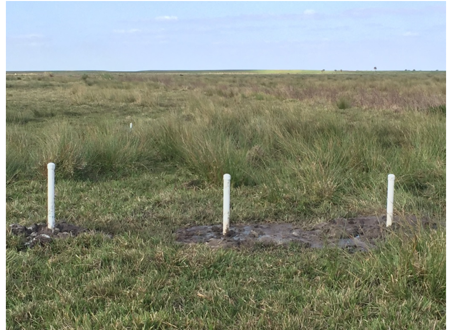
Installed piezometers near SPT boring TB-9
