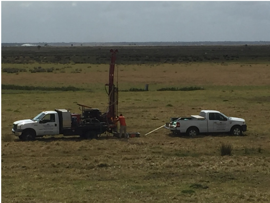
Typical view of interior of site. Drilling SPT borings.
