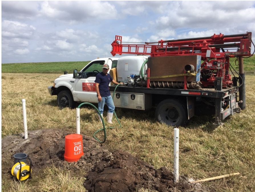
Field permeability testing near SPT boring TB-5
