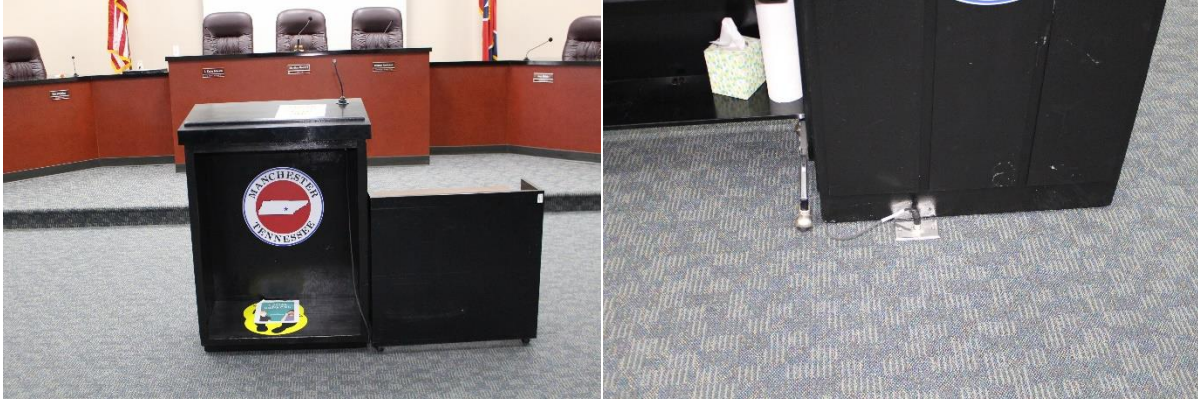
Podium in the Center towards the Front of the Boardroom with One Gooseneck Microphone and Audio Connection in Floor
