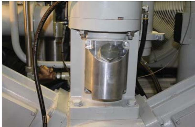
**Figure 34.** Refilling Compressor Crankcase
