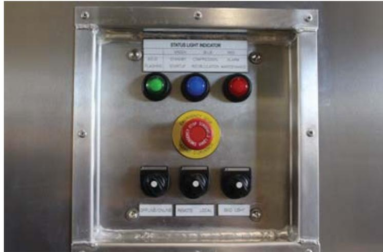
**Figure 11.** Control panel: Online/Offline Switch, ESD button, and Operation Status Lights
