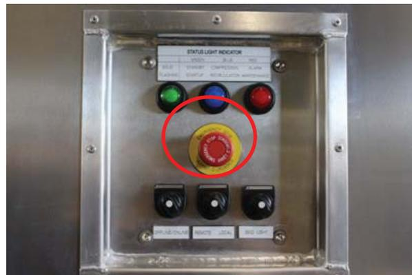
*Figure 14b. ESD Button – Red push button, middle center of panel*
