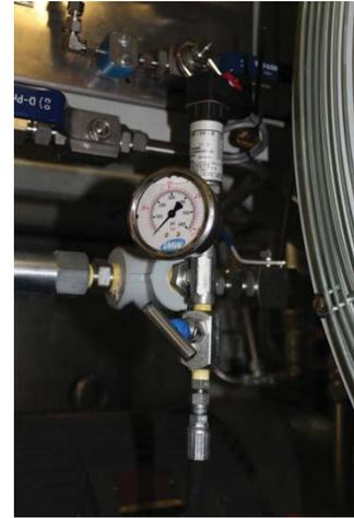
*Figure 23 Pressure Transmitter*
