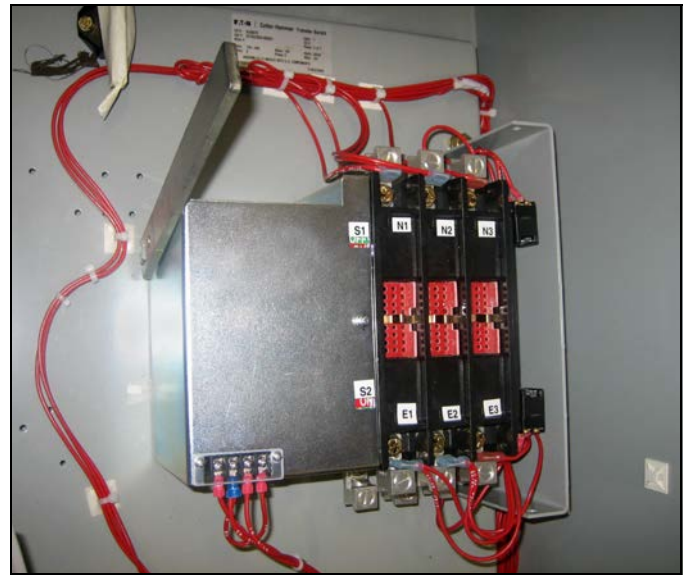
Figure 22. ATS Manual Operating Handle in Use.
