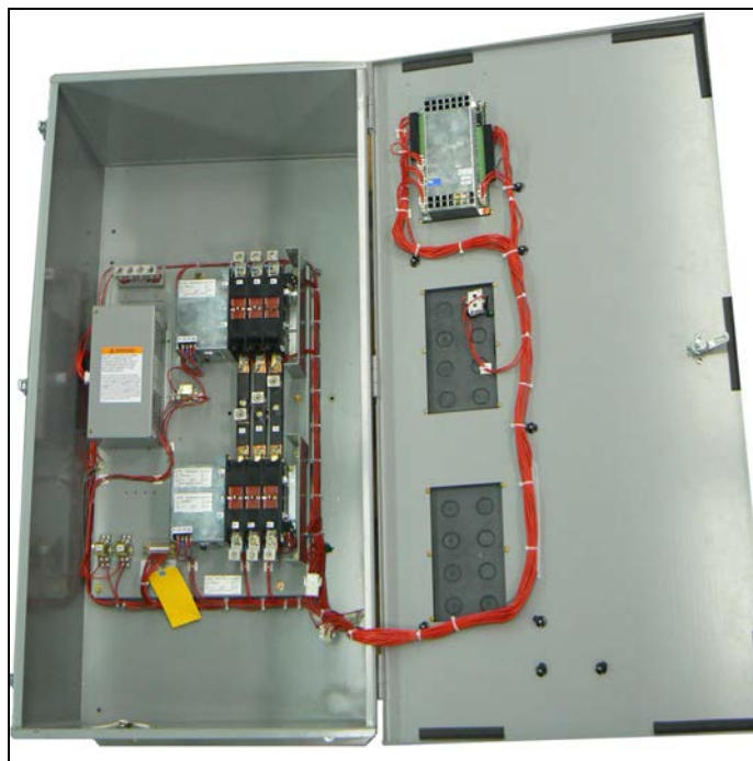
Figure 14. Typical (40A-400A) Closed Transition Contactor Based ATS Equipment (Door Open).
