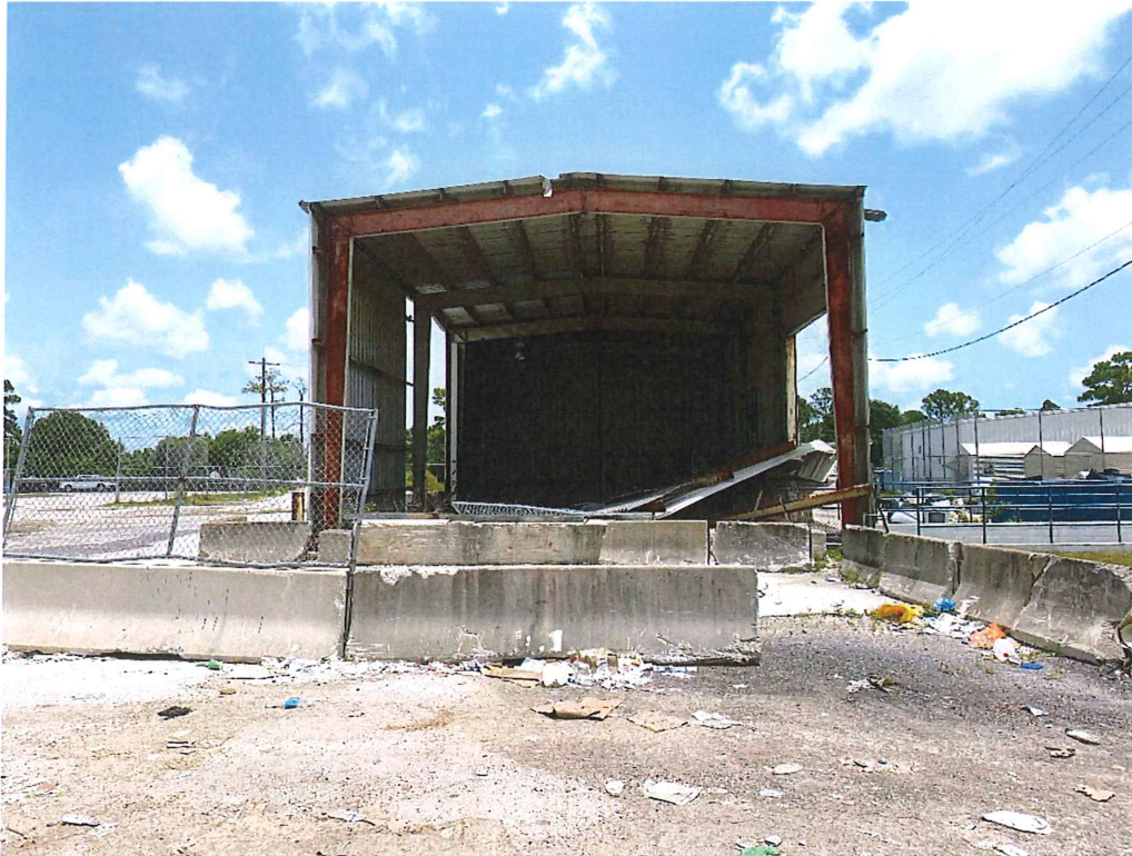
Looking North at Metal Structure
