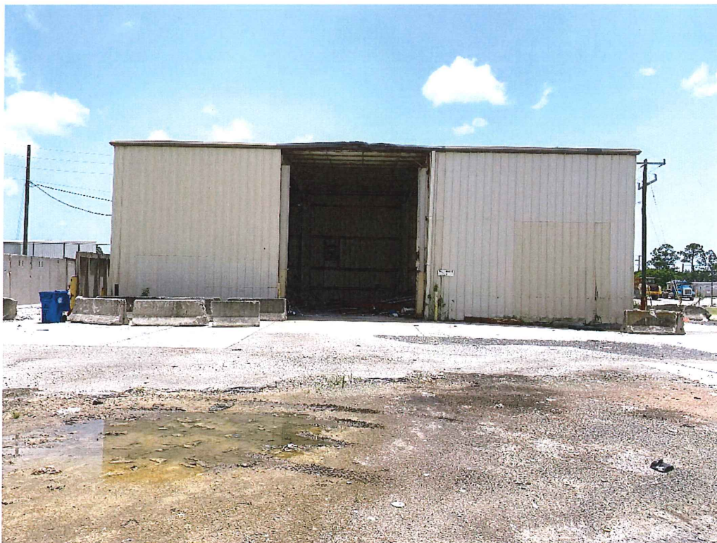
Looking East at Metal Structure
