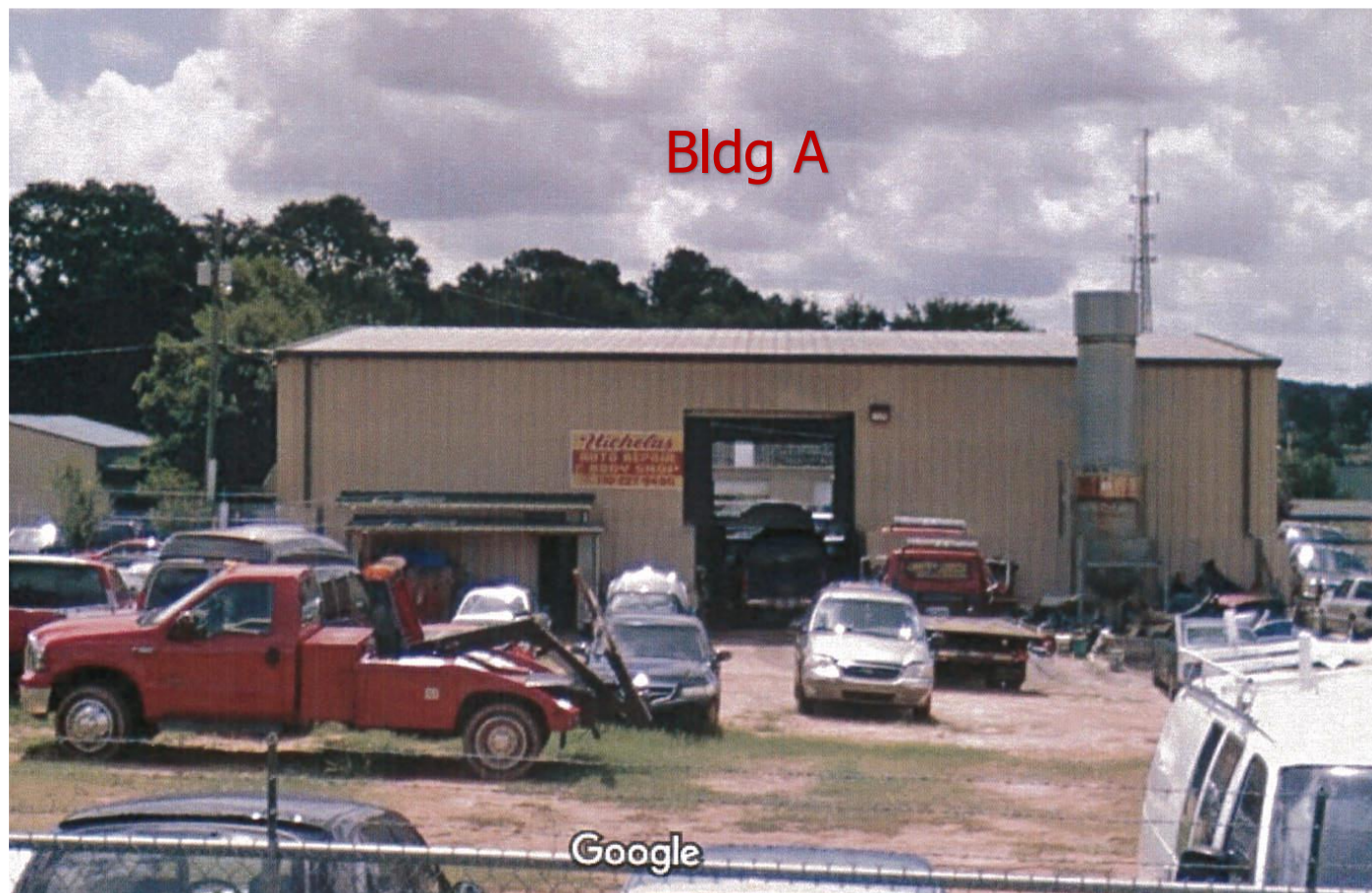
Back of Building A
