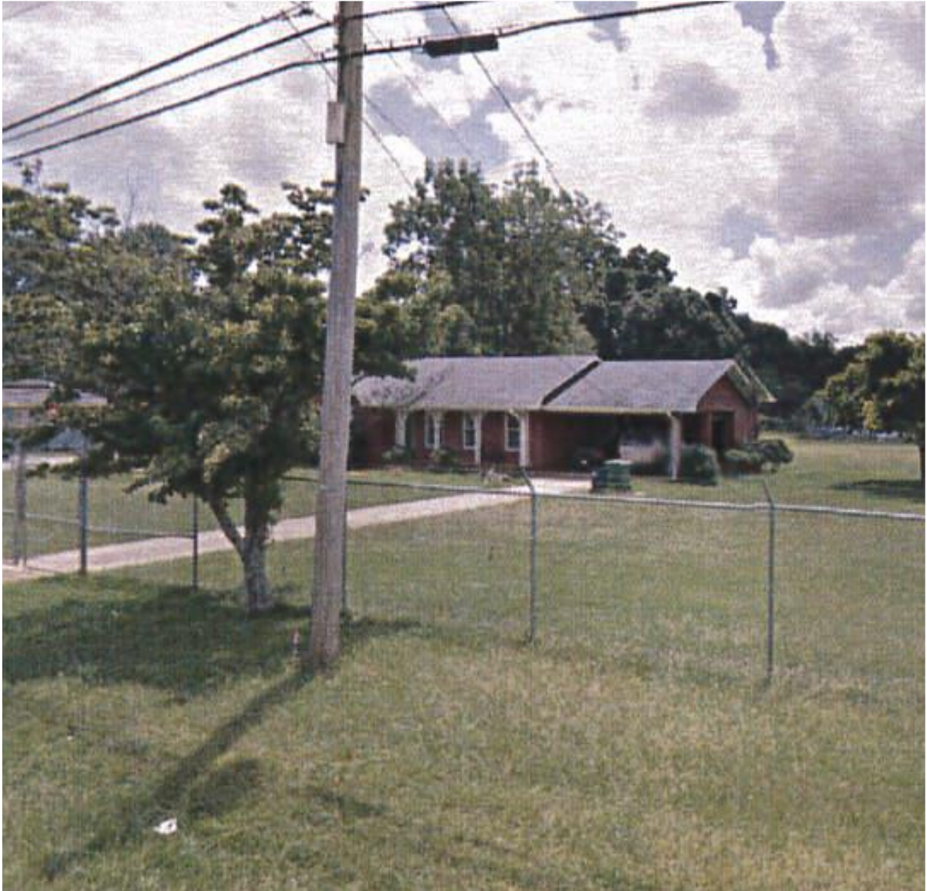
Front of house to be demolished
