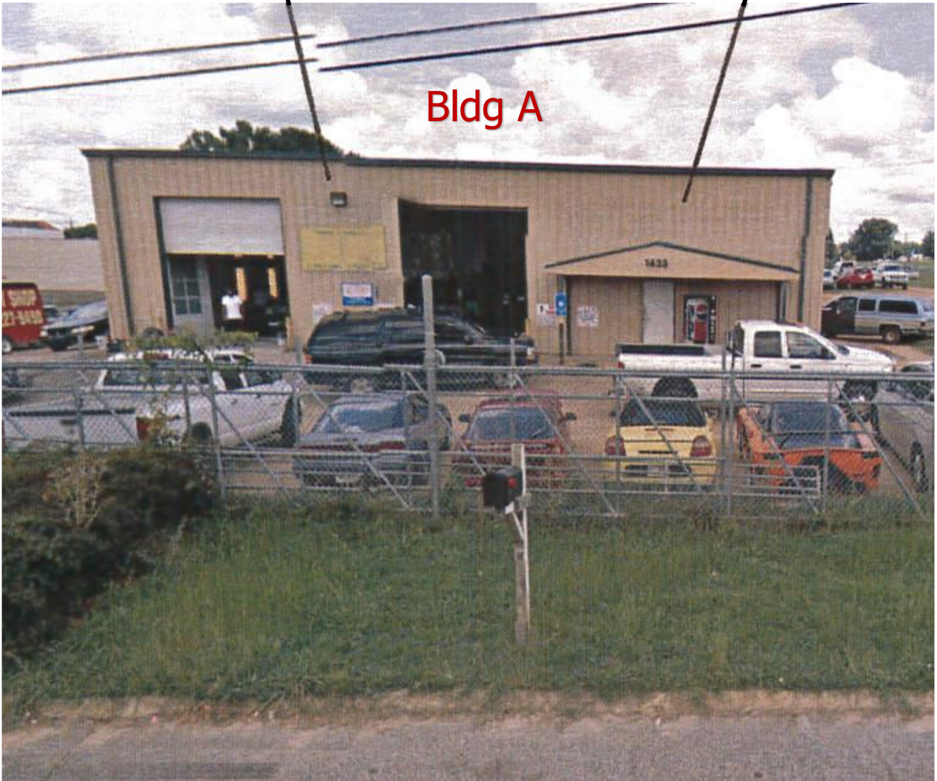
Front of Building A
