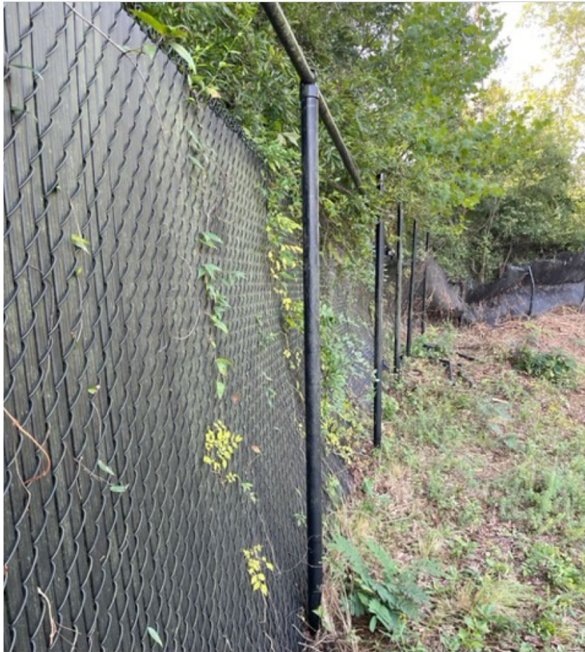
Existing Fence Condition
