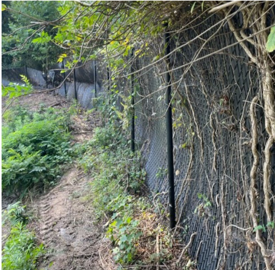
Existing Fence Condition
