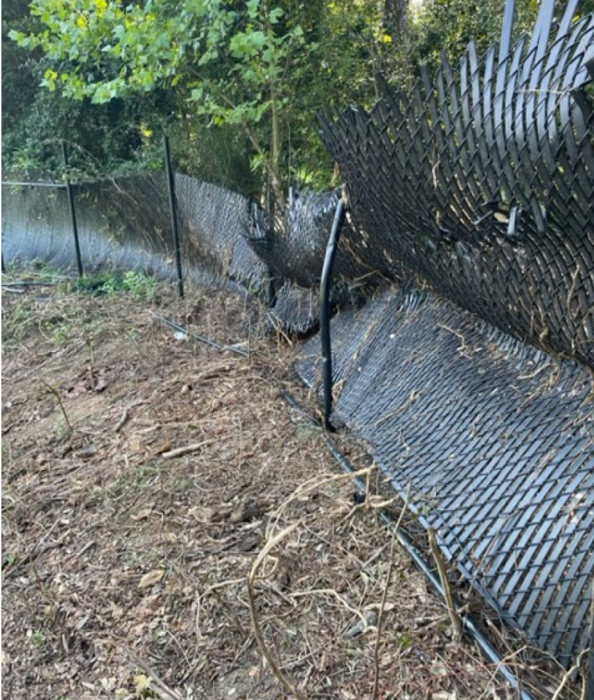
Existing Fence Condition
