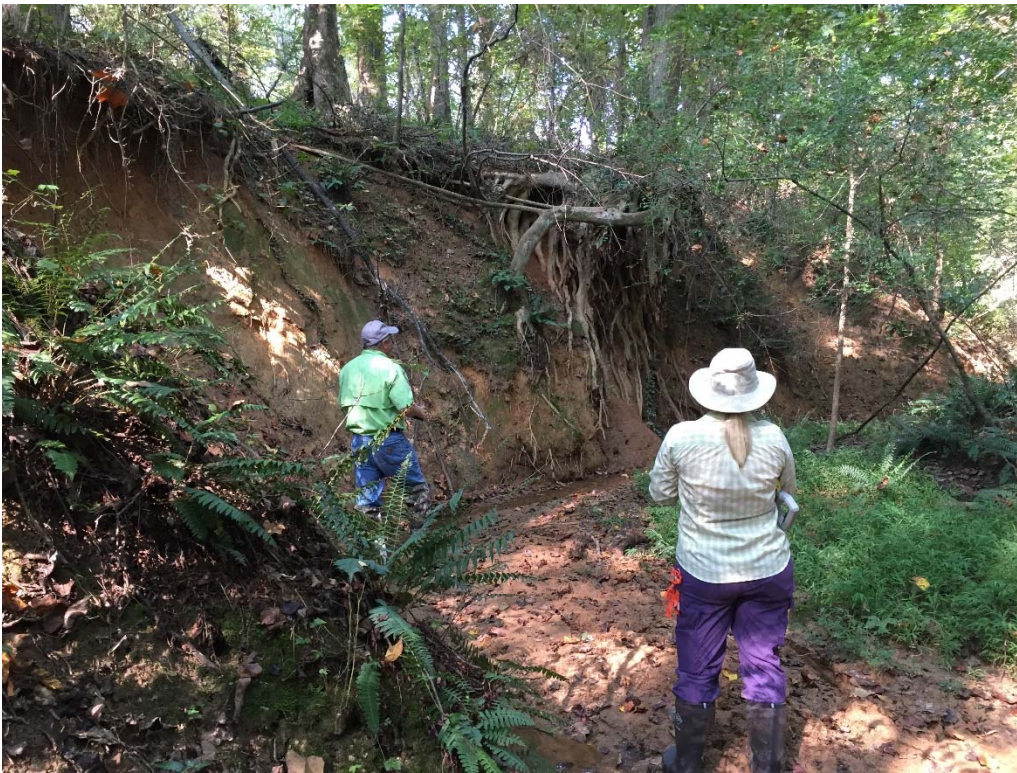
Reach 7 Typical Condition at Upstream End.
