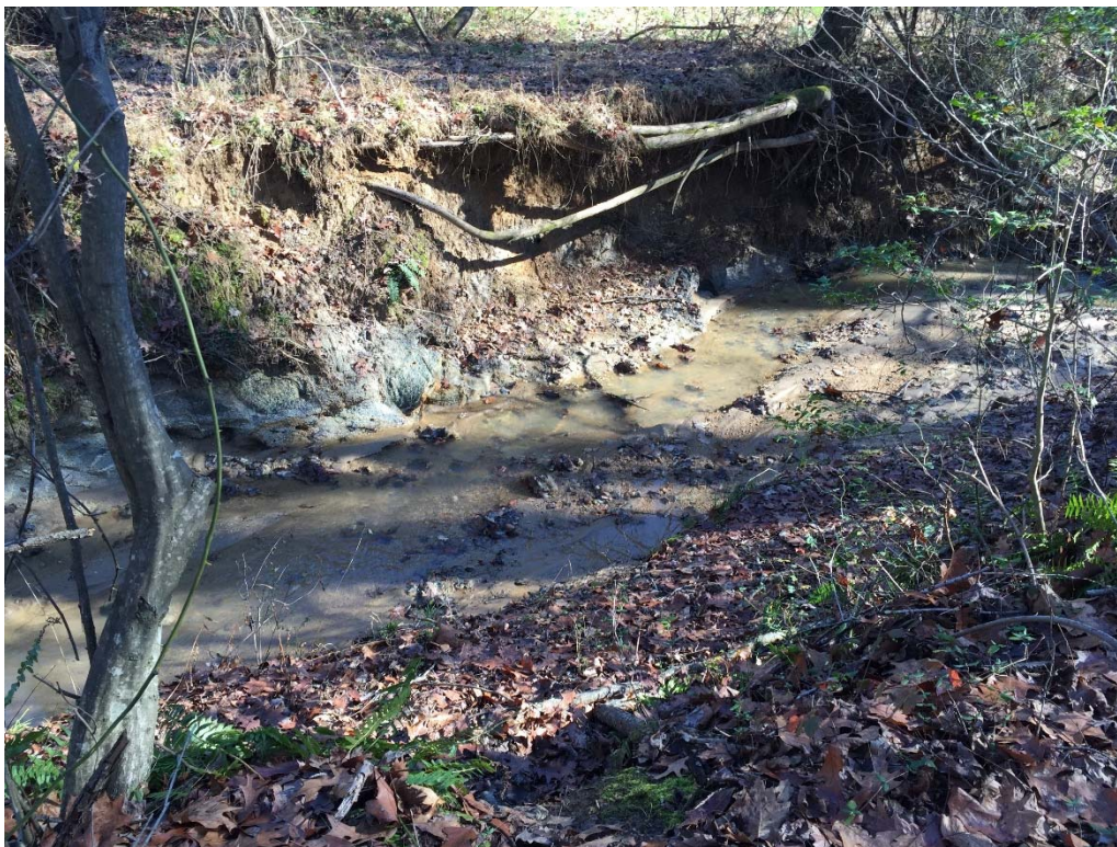
Reach 4 Typical Condition at Downstream End.
