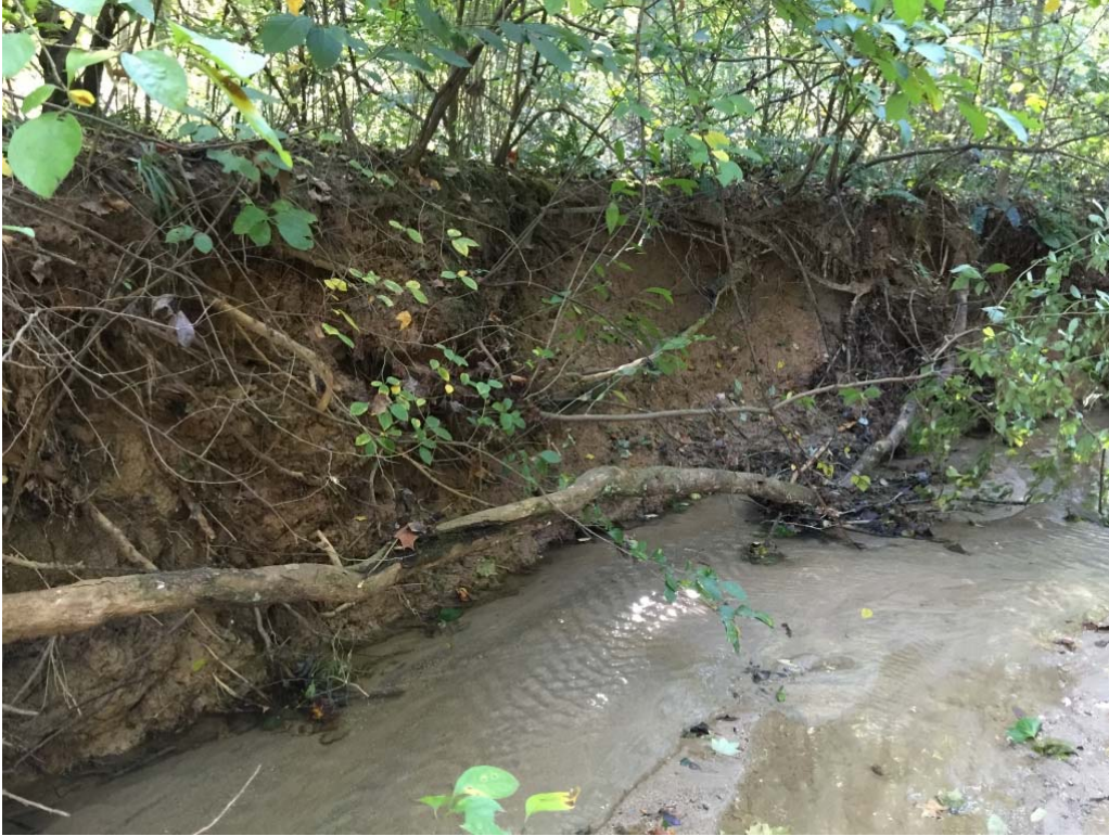
Reach 5 Typical Condition.
