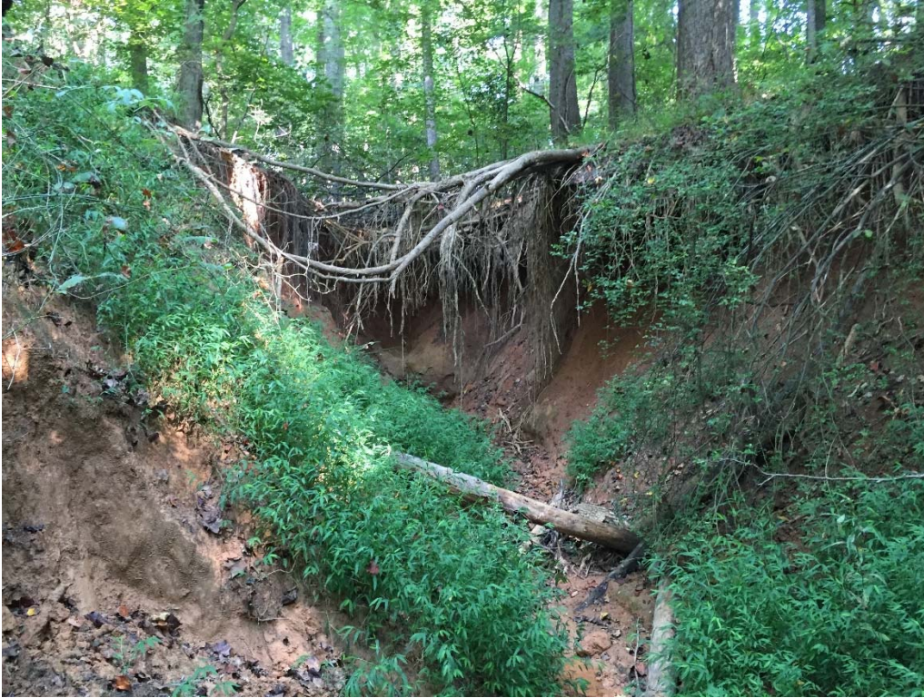
Reach 7 Head Cut at Upstream End.
