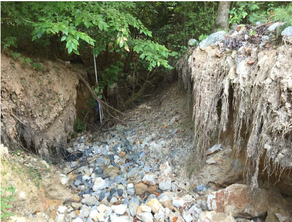
Reach 6 Side Channel Head Cut.
