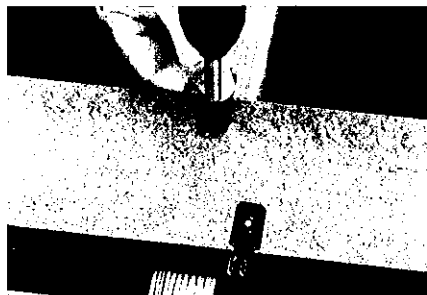
Hidden Fastener Installation to Bottom Surface of Board
