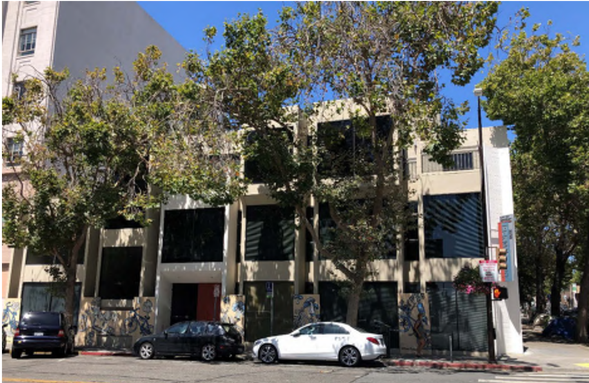
Figure 5 2118 Milvia Way, South Elevation, Facing North
