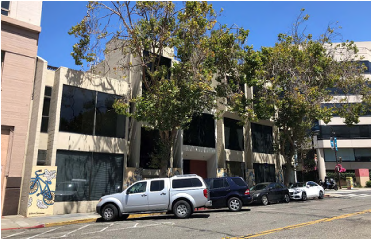
Photo 1. View of project site looking northeast from across Center Street.
