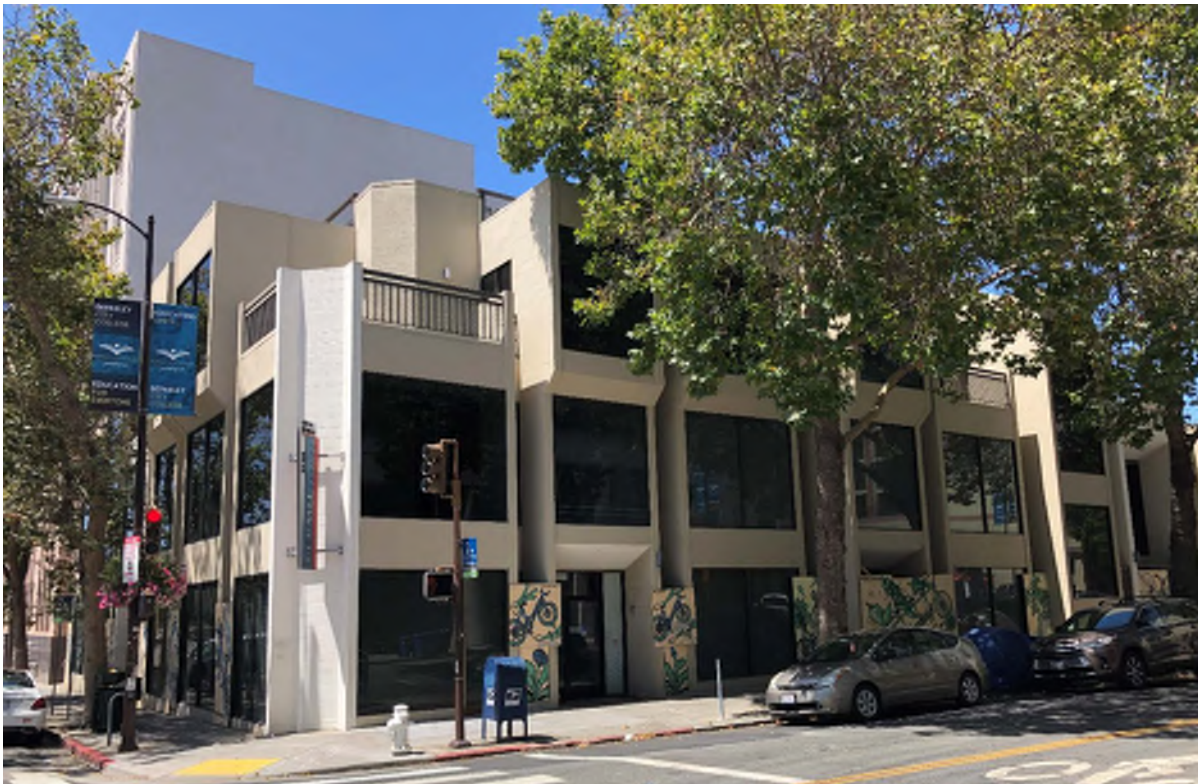
Figure 4 2118 Milvia Street, South and East Elevations, Facing Northwest
