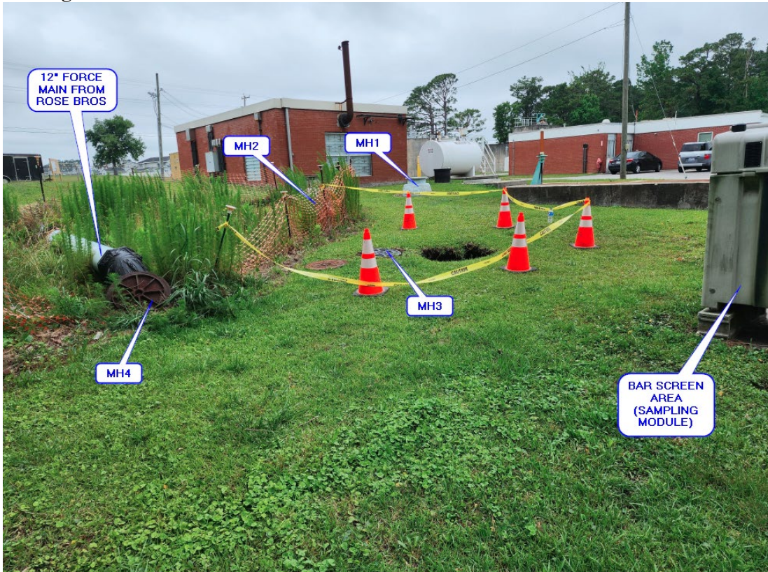
Existing Conditions: view to north.
