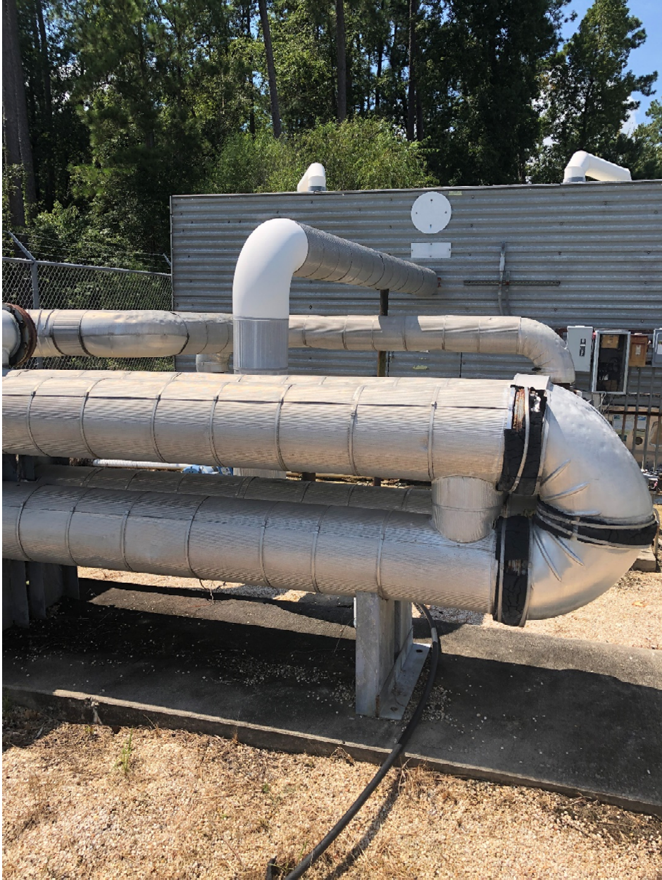
Tower and Heat Exchanger to be removed.
