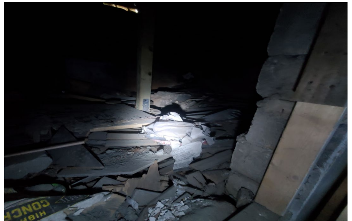
Photo 4 – Original wall material from walls is in piles on basement floor.
