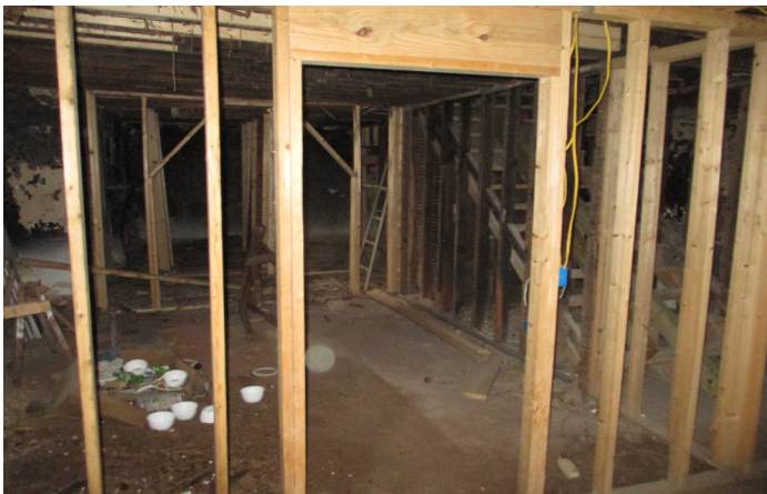
Photo 3 – View of basement from the 2021 assessment.
