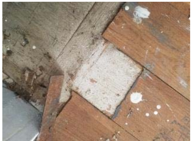
Photo 6 – Wood flooring and vinyl planks.
