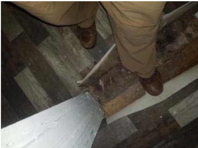
Photo 5 – Multi-layers of vinyl flooring.
