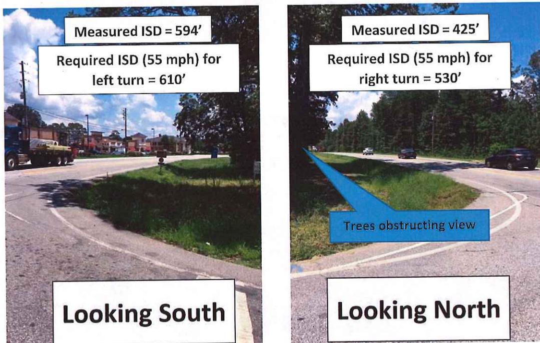
Figure 7. Views of SR-53 and New Cut/Ednaville Road Intersection from Ednaville Road Approach
