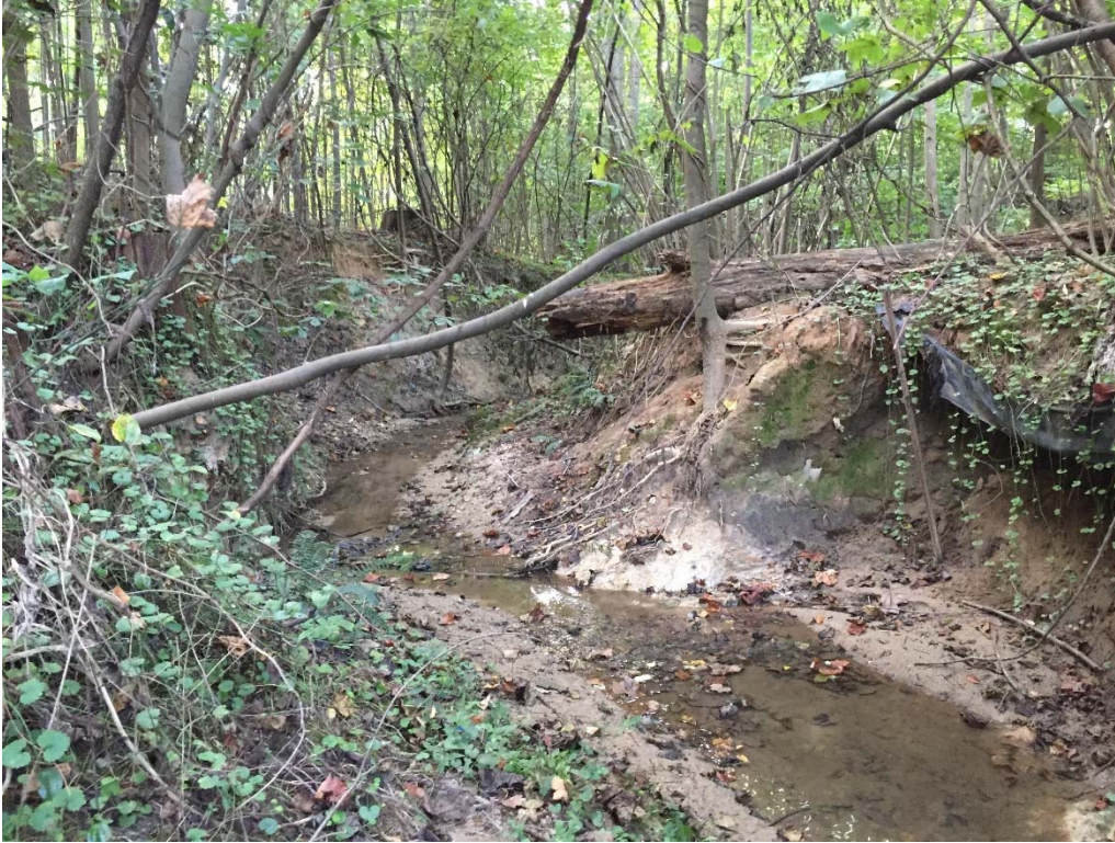
Reach 6 Typical Condition at Downstream End.
