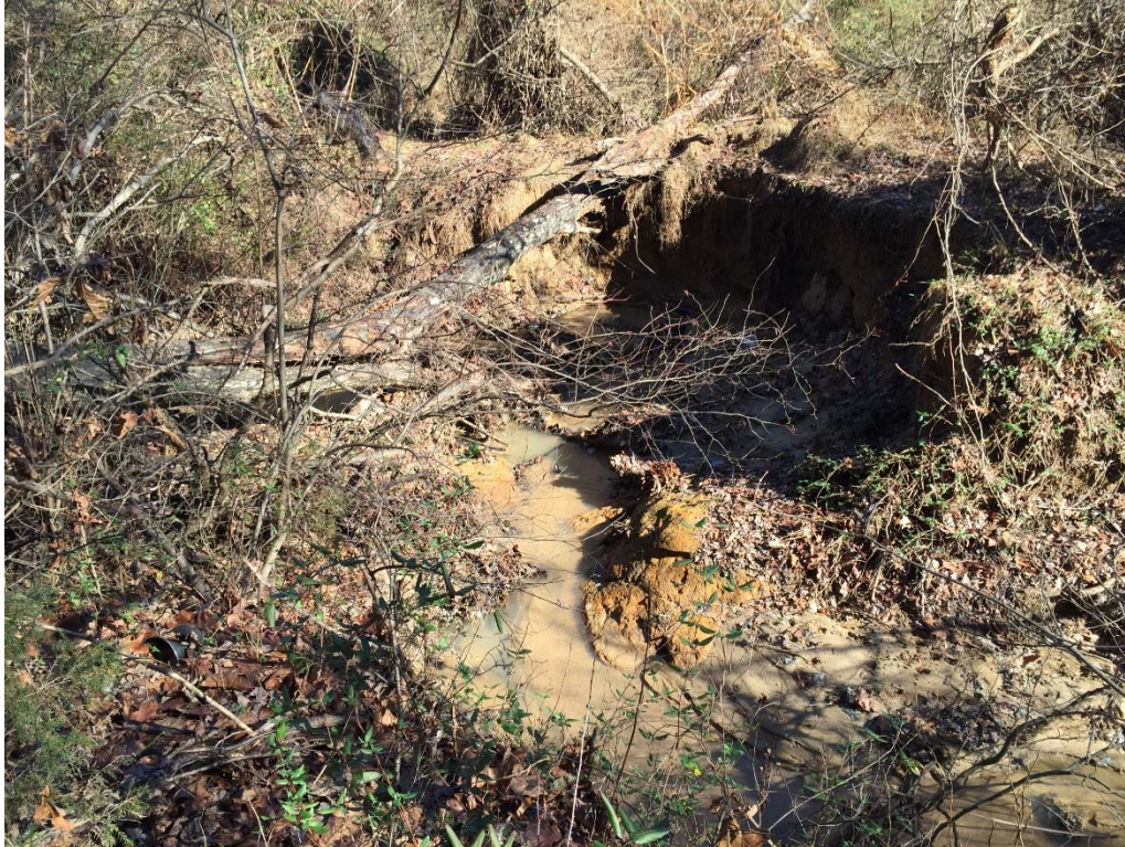
Reach 4 Typical Condition Near Sewer Line.
