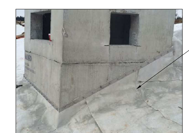
1 DETAIL: GCL CONNECTION TO CONCRETE STRUCTURES AND SLABS NOT TO SCALE
