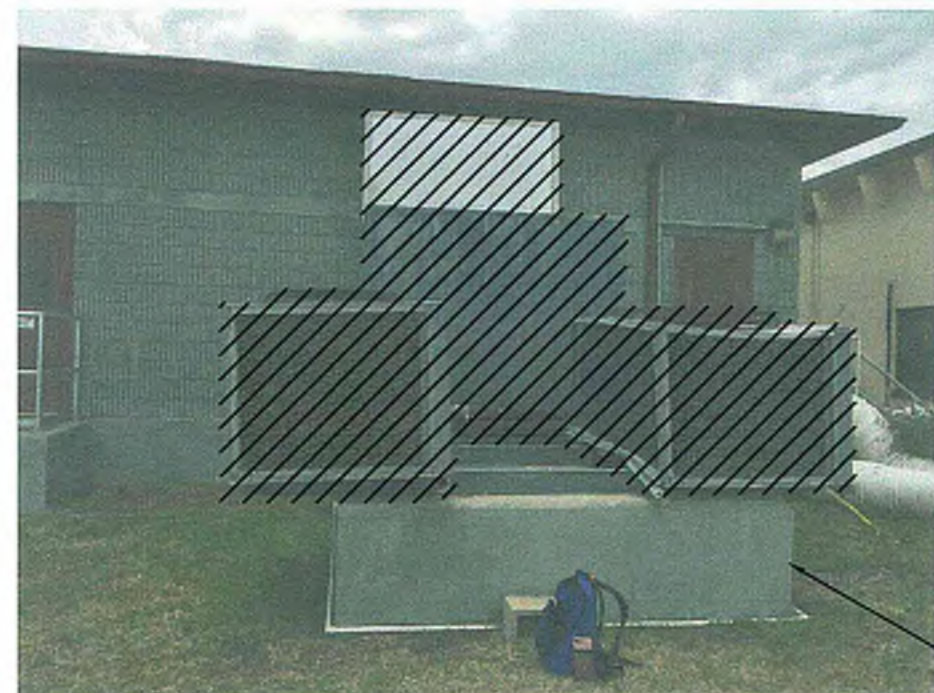
DEMOLITION PHOTO #1 SCALE: NO SCALE
