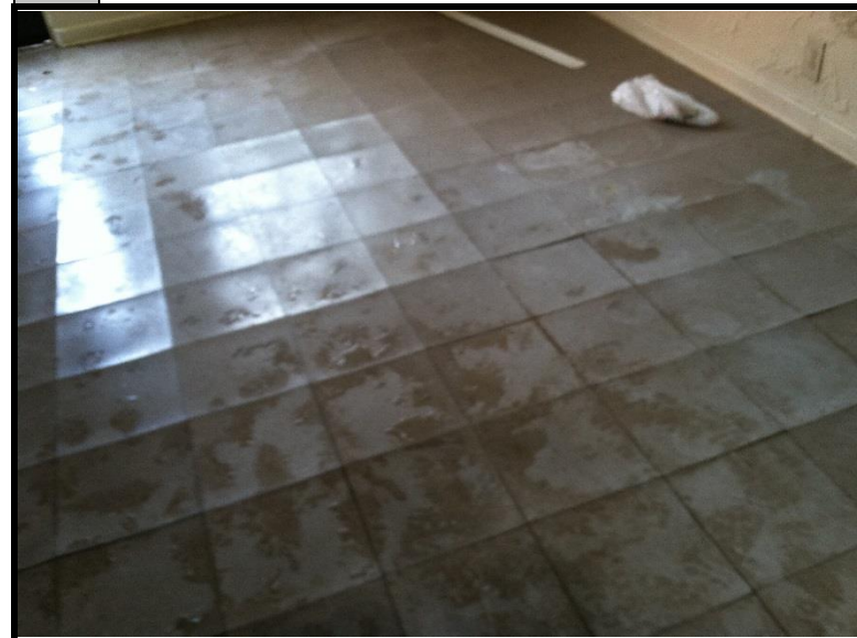
8 General view of floor tile
