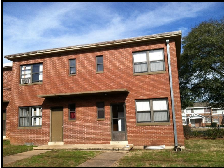
1 General Building view
