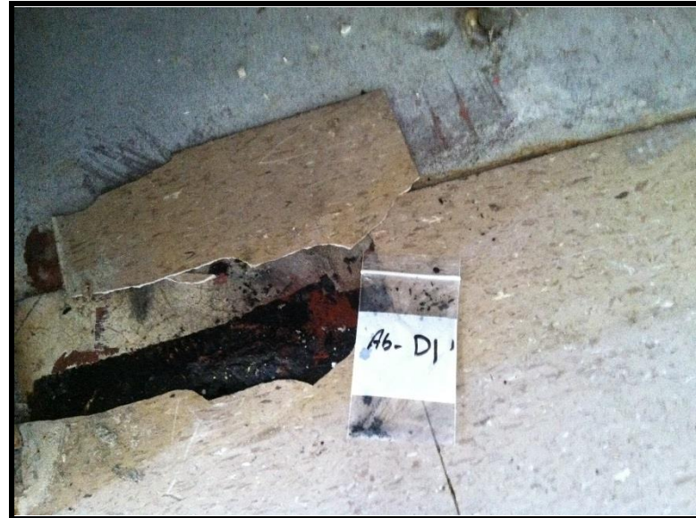
6 Floor tile and black mastic Sample D – no asbestos
