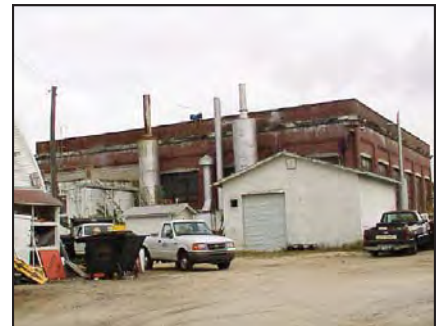
Public Works' Powerhouse
