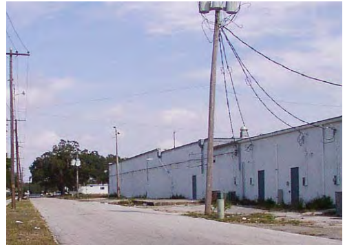
The rear of a shopping center facing N. Ridgewood abuts a residential neighborhood.
