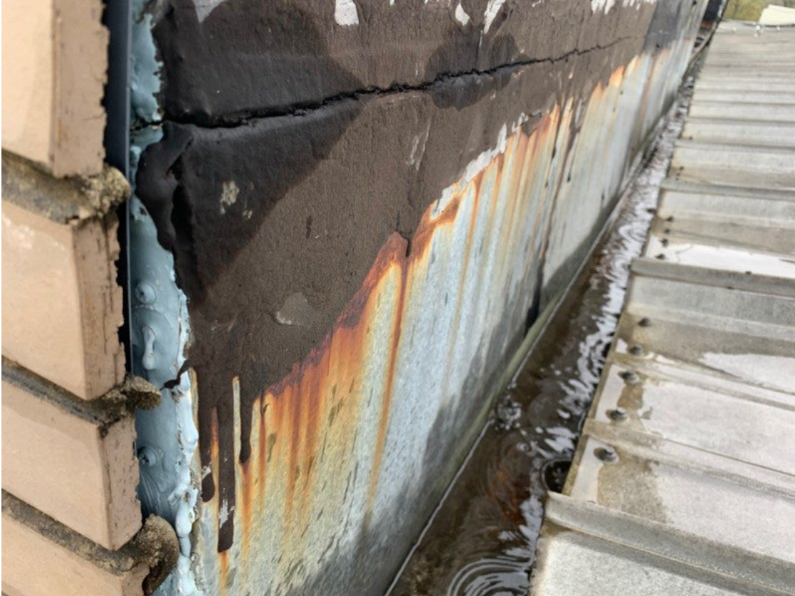
Gutter and Parapet Wall
