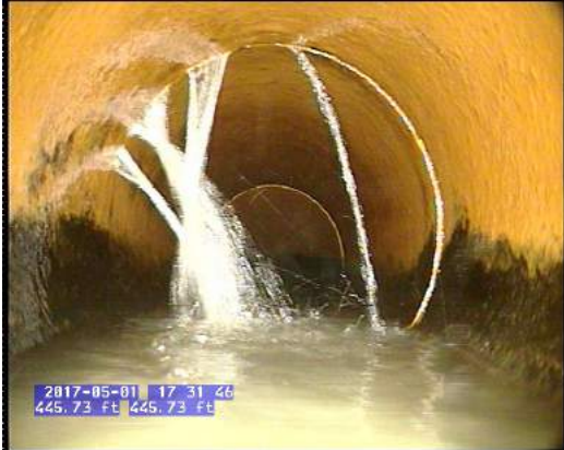
P36 P74 (2)_1d7db7c9-9892-4522-b16b-7c32cfc485b6.bmp, 00:09:07, 445.83 Infiltration Gusher, at 12 o'clock
