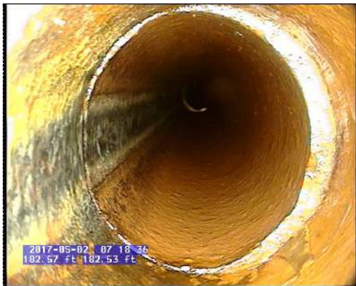
P37 P36_b7094d30-0d4d-454a-88c2-8114f941e086.bmp, 00:05:55, 182.61 Tap Factory Made, at 9 o'clock, 4 inch dim
