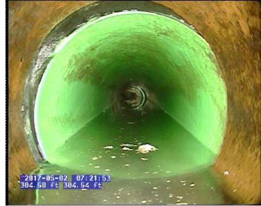
P37 P36_353786e2-1fe4-41bd-b20f-ac543e8f9d10.bmp, 00:08:40, 304.66 Infiltration Runner, at 11 o'clock
