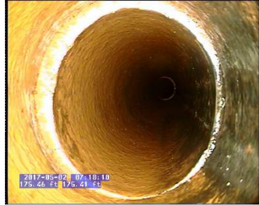
P37 P36_7e6232c3-7cf3-427c-9535-e85cba75259d.bmp, 00:05:36, 175.49 Tap Factory Made, at 3 o'clock, 4 inch dim
