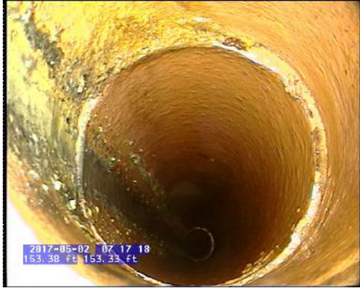
P37 P36_81c10840-7713-459b-a284-64e64fec1ddc.bmp, 00:04:52, 153.41 Tap Factory Made, at 9 o'clock, 4 inch dim
