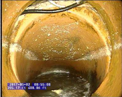
P86 P36_6c59f69c-2e0f-43af-9dd0-b94bcb7fe39a.bmp, 00:05:23, 285.24 Joint Offset Large, 0 ° displacement
