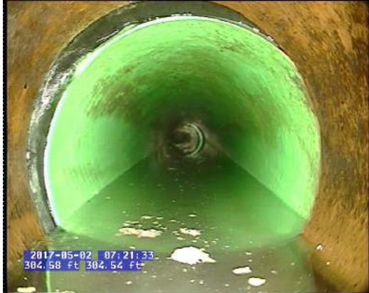
P37 P36_96f667c2-ef13-41d9-a588-bd7fb5b76af9.bmp, 00:08:36, 304.66 Material Change, Polyvinyl chloride
