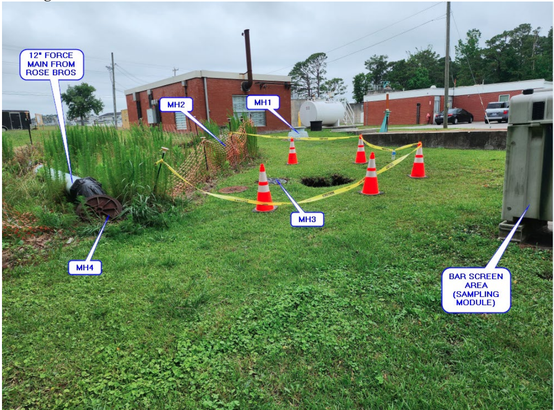
Existing Conditions: view to north.
