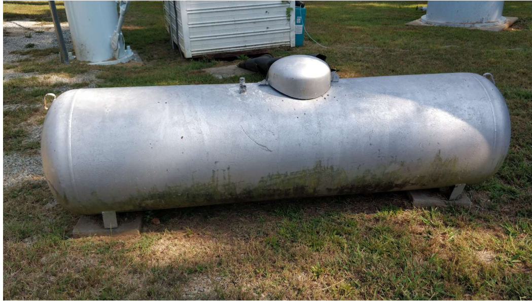
Figure 4.7.2.B - Fuel tank shows rust
