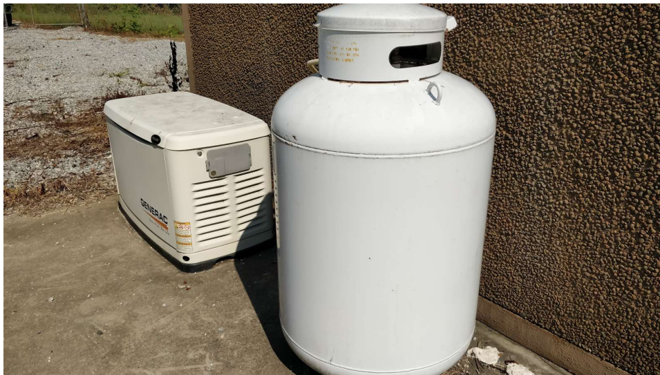
Figure 4.8.2.A - Generator and Fuel tank undersized and not secured
