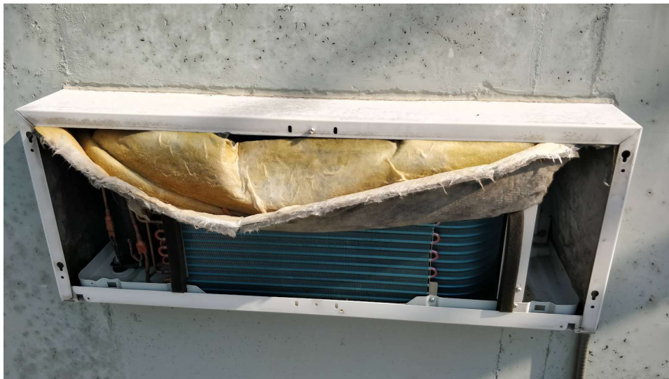
Figure 4.6.2.E - HVAC unit cover is off and insulation falling out
