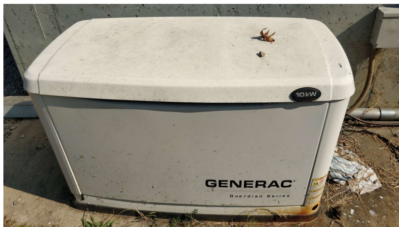
Figure 4.7.2.A - Generator case rusted and not secured to ground
