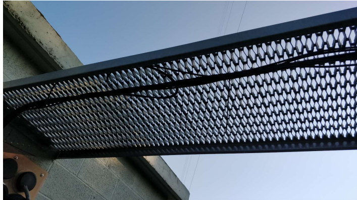
Figure 4.3.2.D - Cables not secured
