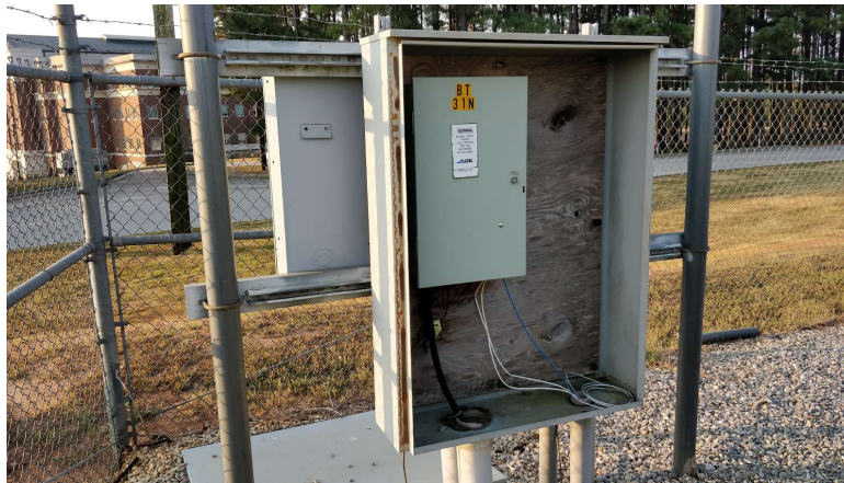
Figure 4.2.1.B - Fiber connection box
