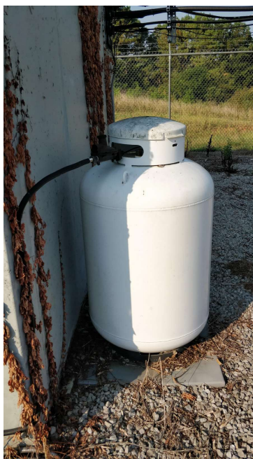
Figure 4.4.2.B - Fuel tank not secured or grounded
