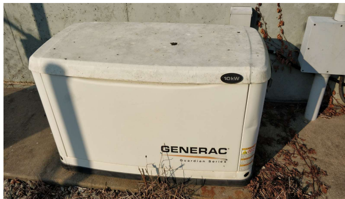
Figure 4.4.2.A - Generator undersized and not secured
