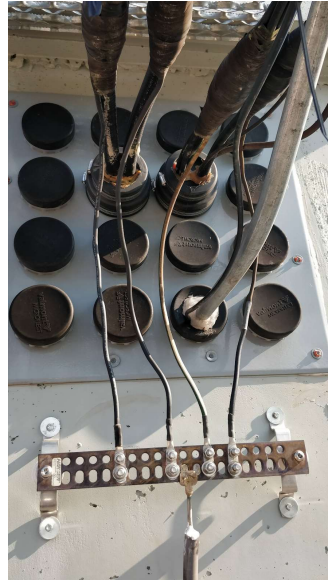
Figure 4.5.2.B - Rigid conduit incorrectly sealed through the window
