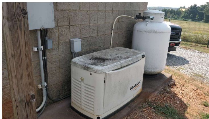
Figure 4.9.2.A - Generator and fuel tank
