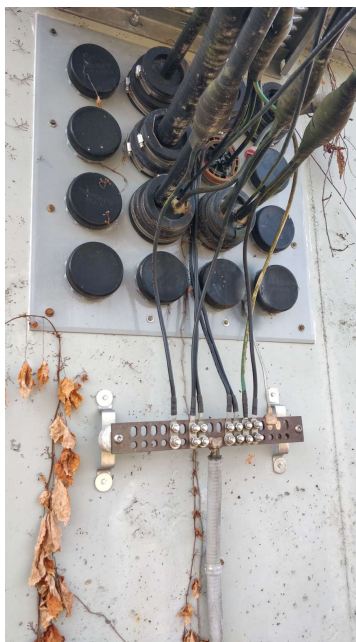
Figure 4.4.2.C - Not all coax grounded and missing coax boot
