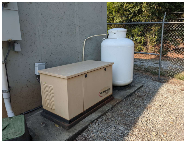
Figure 4.5.2.A - Generator and fuel tank not secured.
