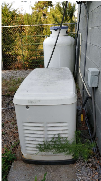
Figure 4.3.2.A - Site generator not mounted down, nor grounded
