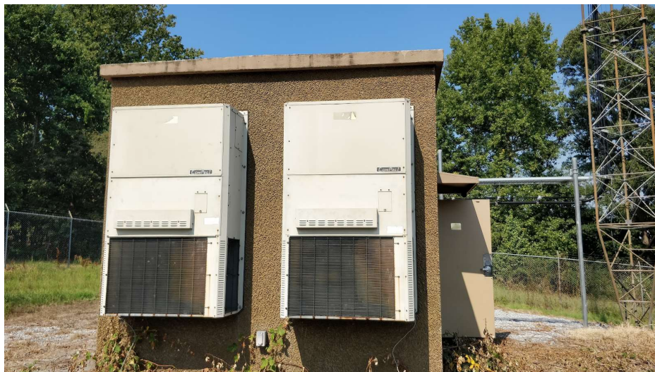
Figure 4.8.2.B - Dual HVAC unit, and appropriate shelter size
