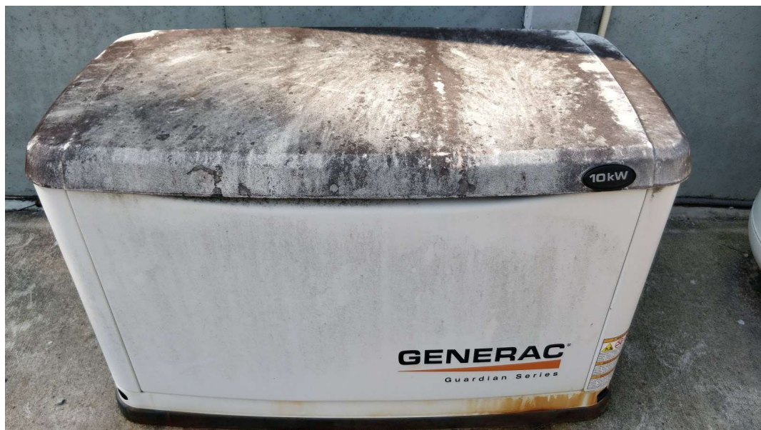
Figure 4.6.2.A - Site Generator not secured
