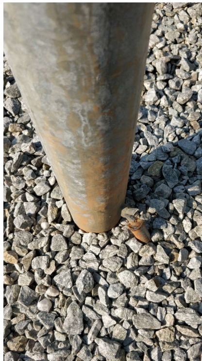
Figure 4.5.2.E - Rusting / Corroding posts
