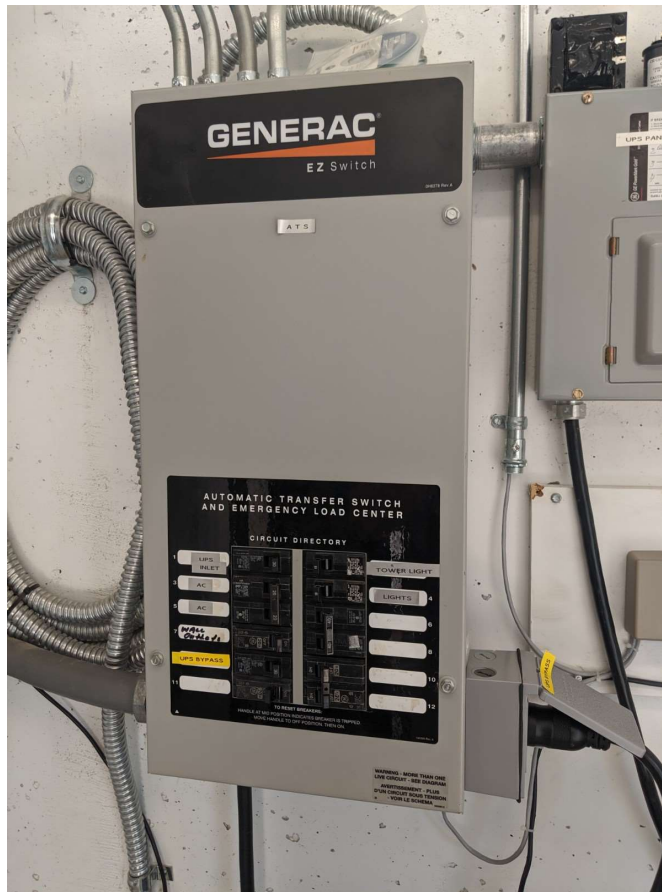
Figure 4.4.1.C - Automatic Transfer switch
