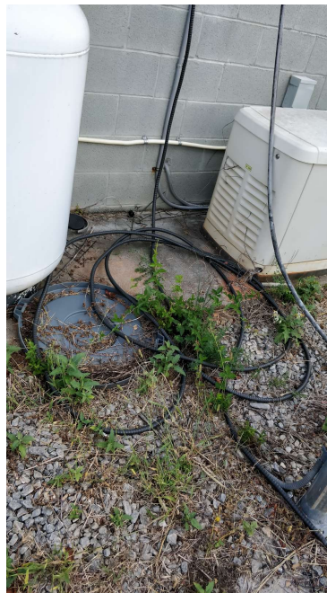
Figure 4.3.2.C - Cables lying on ground
