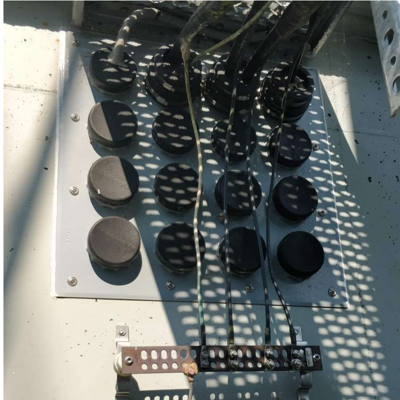
Figure 4.7.2.D - Improperly sealed pass through window (Top left)
