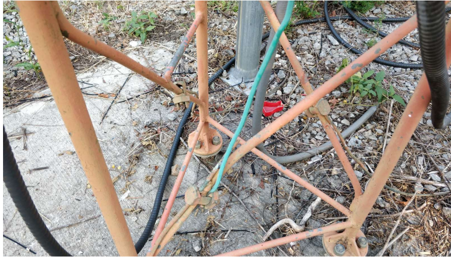
Figure 4.3.2.F - Improper grounding
