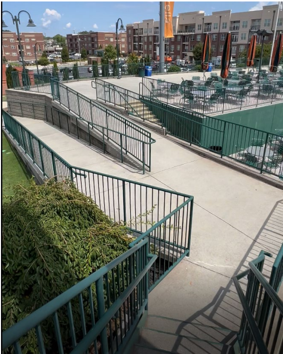
Ramps with wide turn areas.
