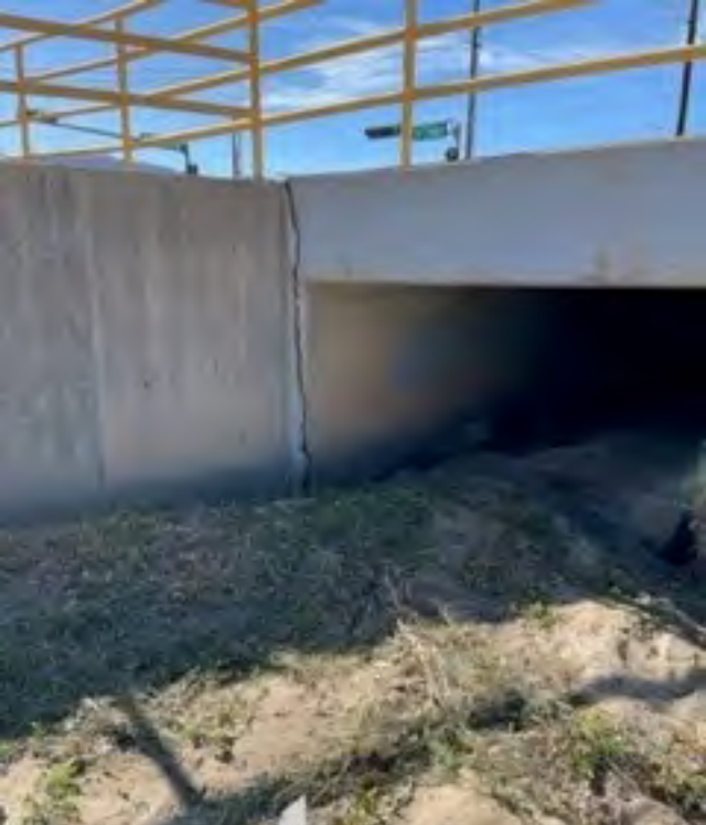
EXHIBIT A - TENTH STREET BRIDGE
