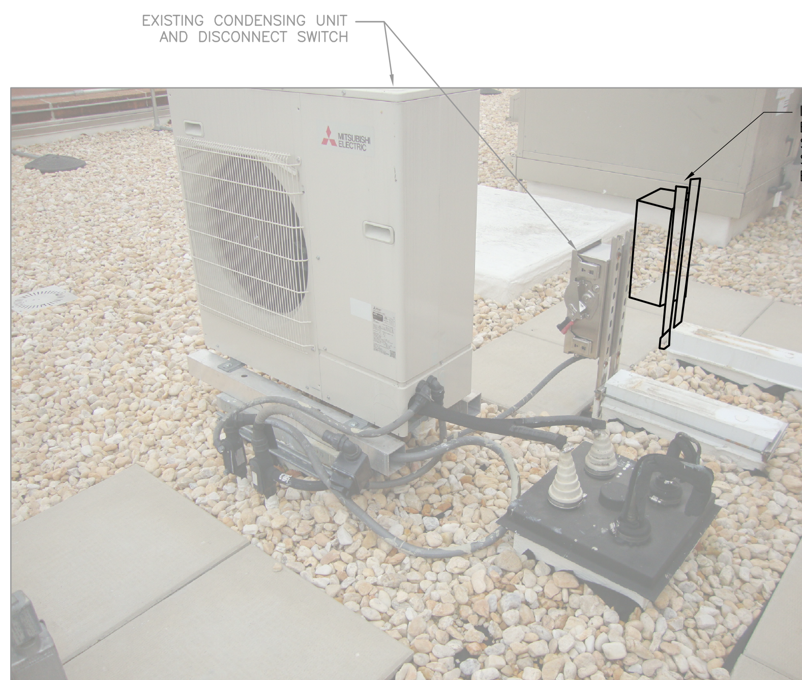
ROOF CONDENSING UNIT DS SECTION 4 NOT TO SCALE E-21
