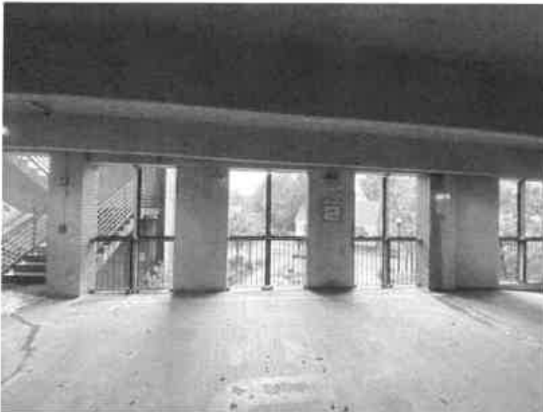
PHOTO 48: BEAM LINE ADJACENT TO STAIRS
