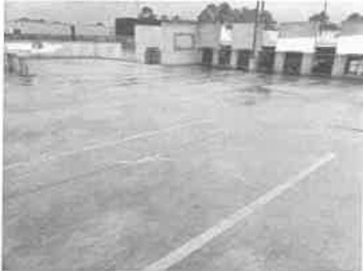
PHOTO 5: OVERVIEW OF UPPER LEVEL DECK
