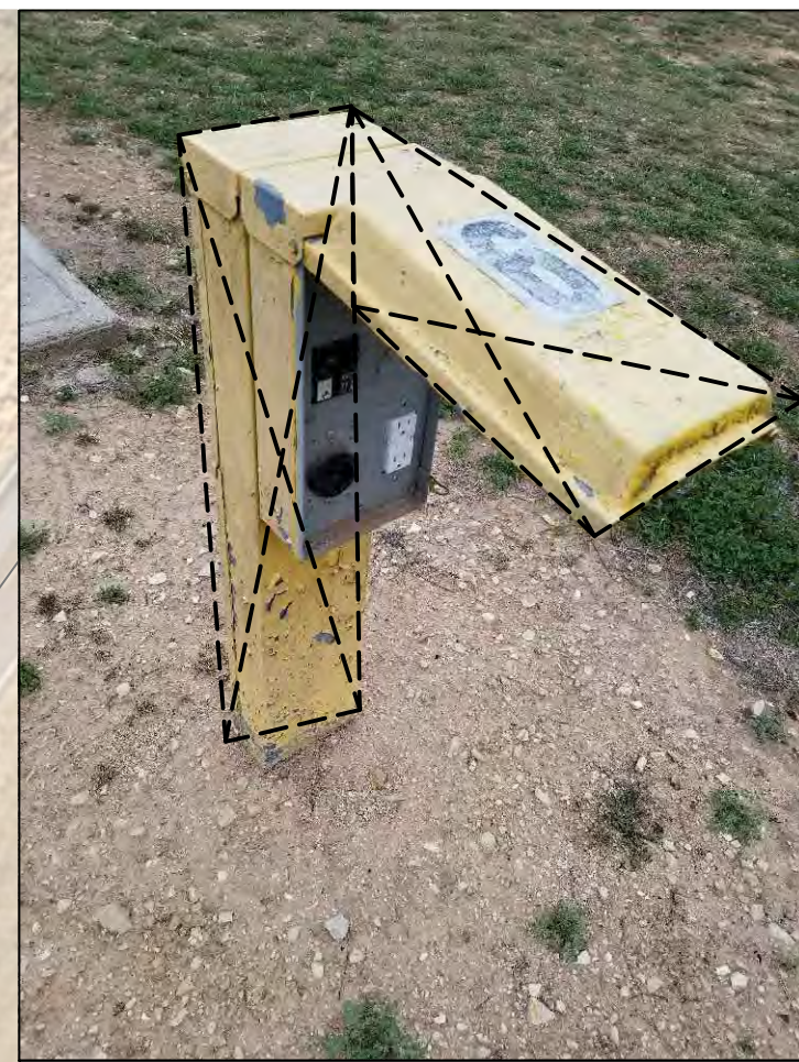
5 PHOTO - DEMOLITION ① E2.0 SCALE: NTS
