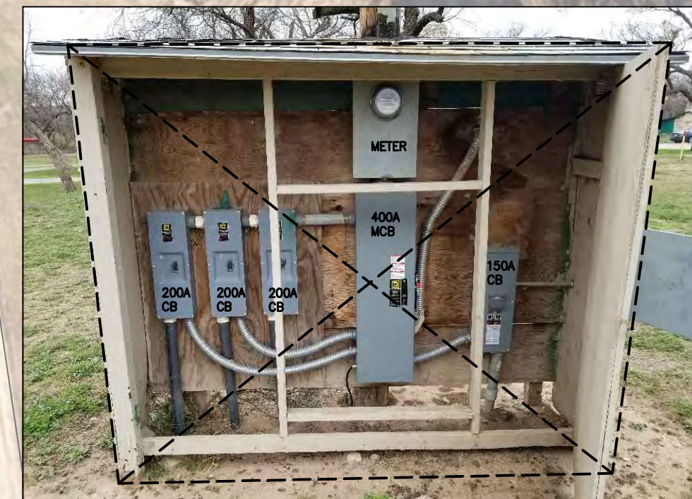
4 PHOTO - DEMOLITION ⑥ E2.0 SCALE: NTS
