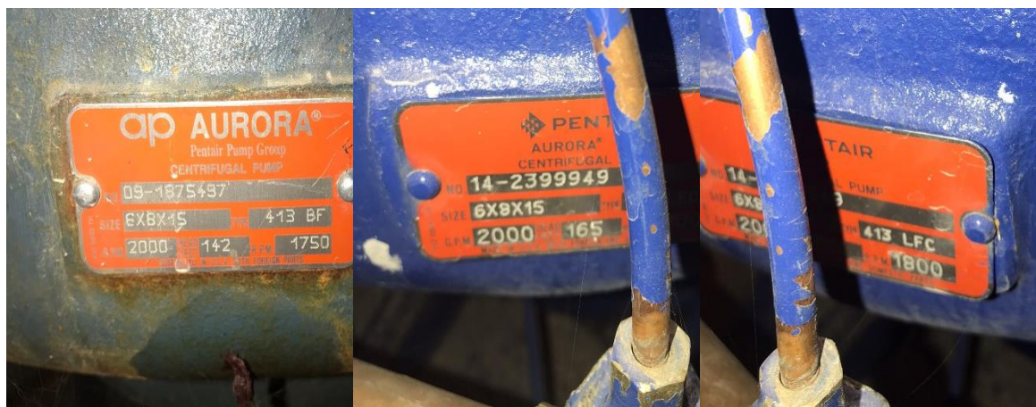
Figure 25 – Pump Nameplates
