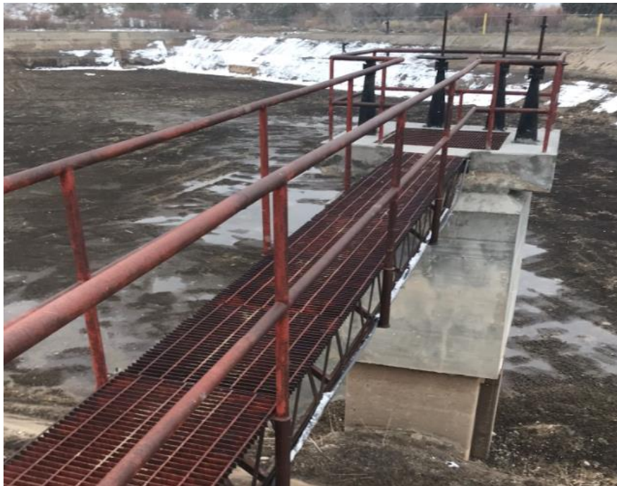
Figure 24 – Minimal Rust of Surface Coating
