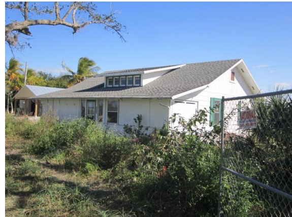
Photo #4 View of building facing northeast.
