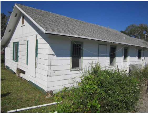
Photo #3 View of building facing northwest.
