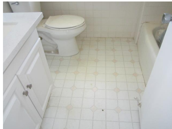
Photo #6 View of off-white & peach "box" pattern SVF reported to be ACM.
