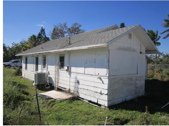
Photo #2 View of building facing southwest.
