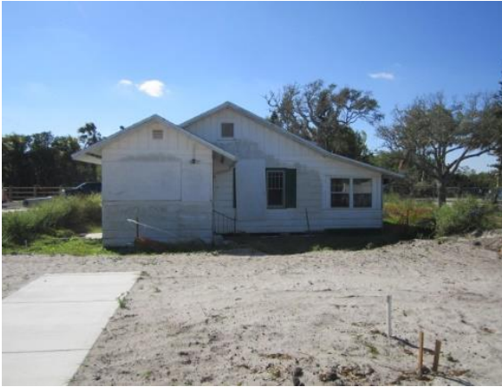
Photo #1 View of building facing south.
