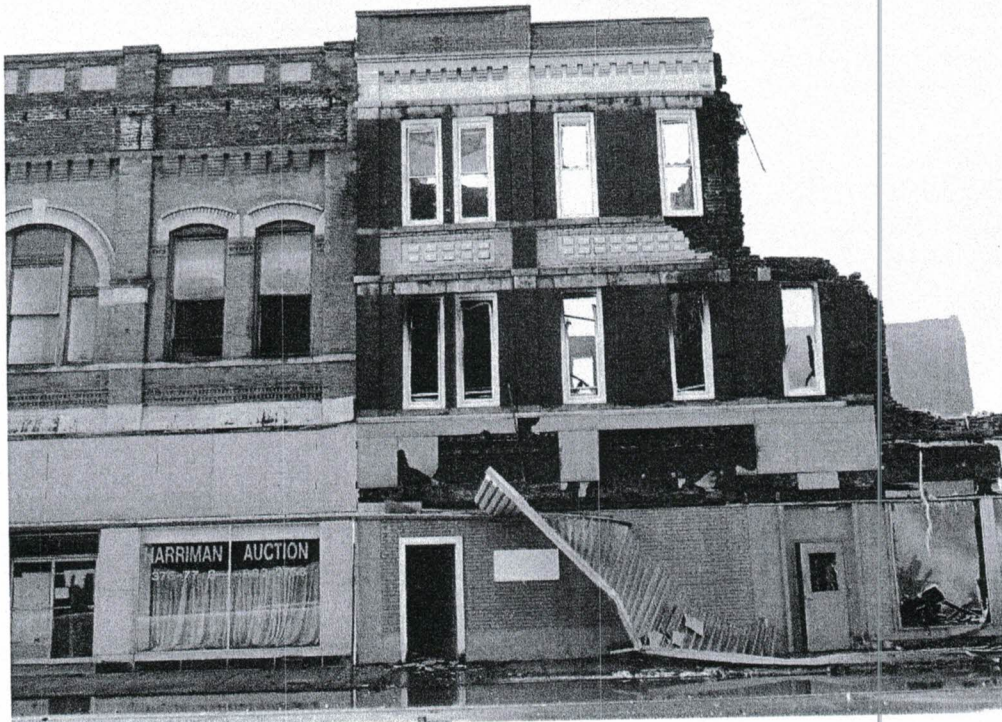
Photograph 2: Remaining portion of the building at 529 North Roane Street.
