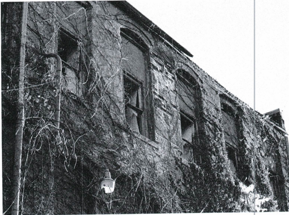
Photograph 8: The top of the southwest corner is leaning outward from the building.
