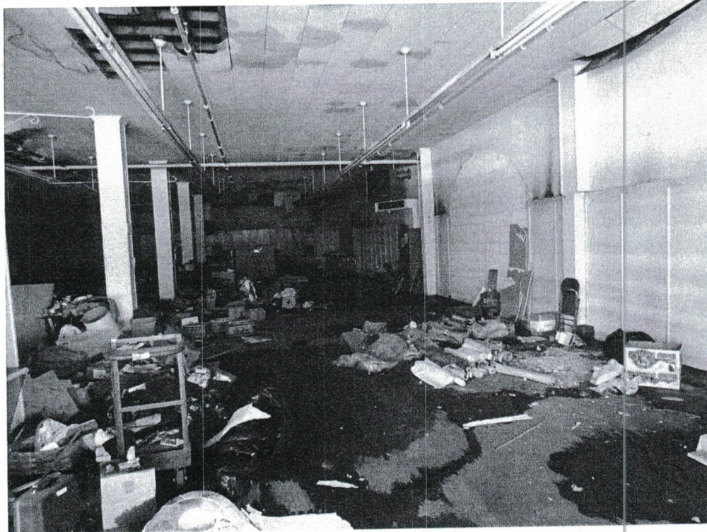
Photograph 12: First floor of building 523 facing west along the north wall.
