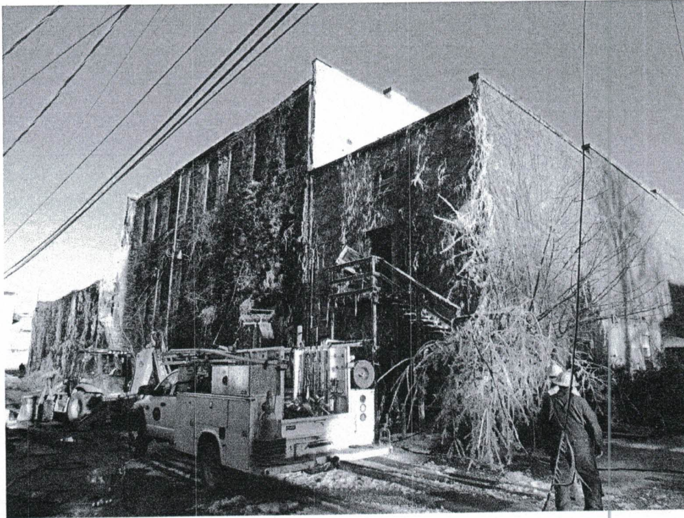
Photograph 5: Southwest corner of the buildings.
