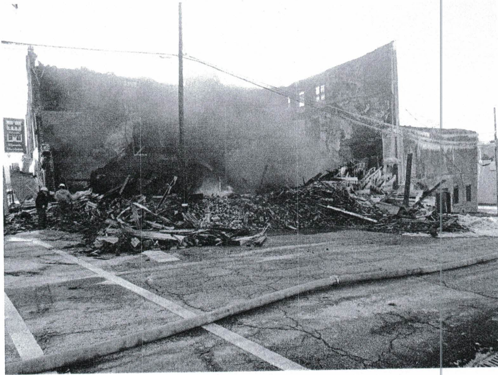
Photograph 1: The northeast corner building has burned and collapsed.
